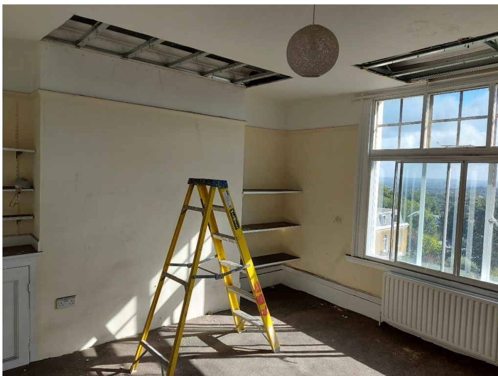
Figure 9: The second floor rear room, showing the suspended ceiling and the metal casement window
