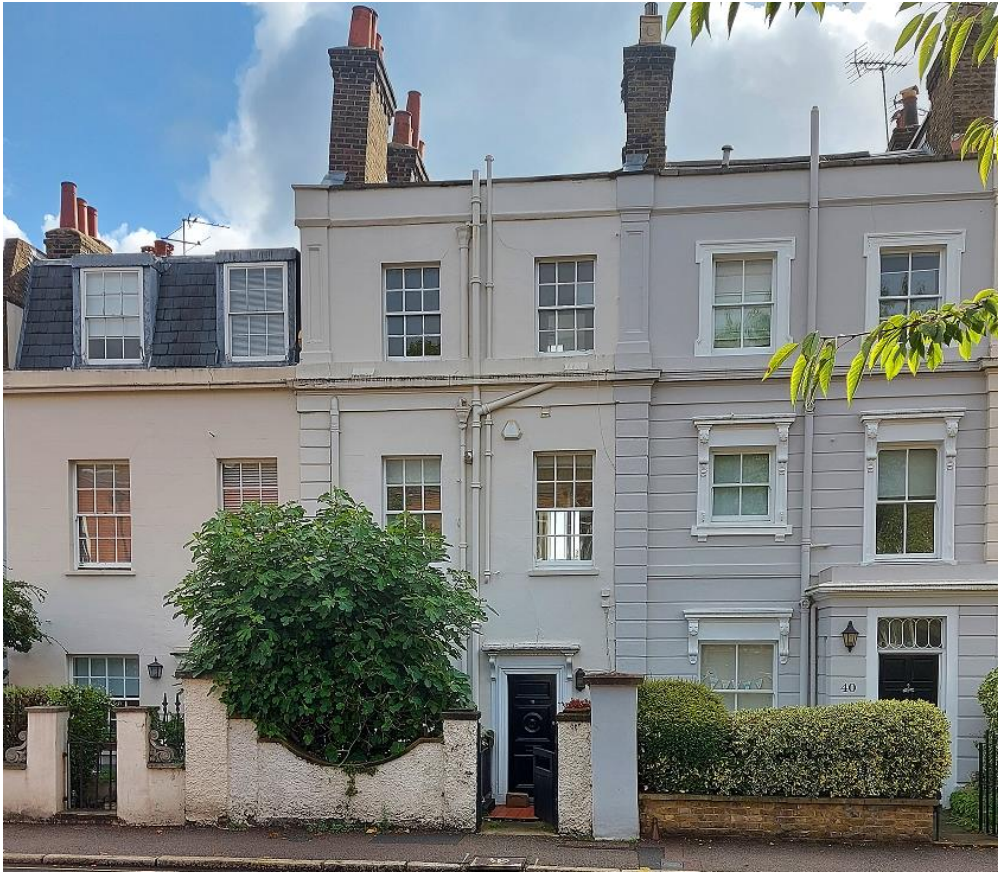
Figure.5: The street front of 42 Southwood Lane
