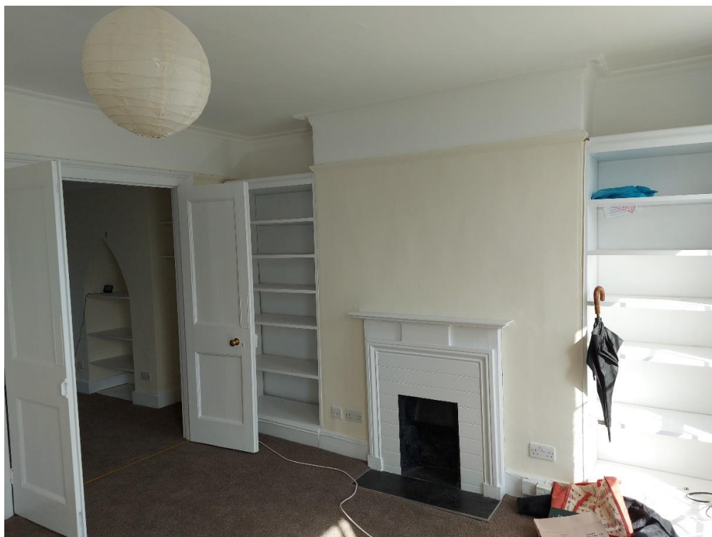
Figure 8: The ground floor rear room
