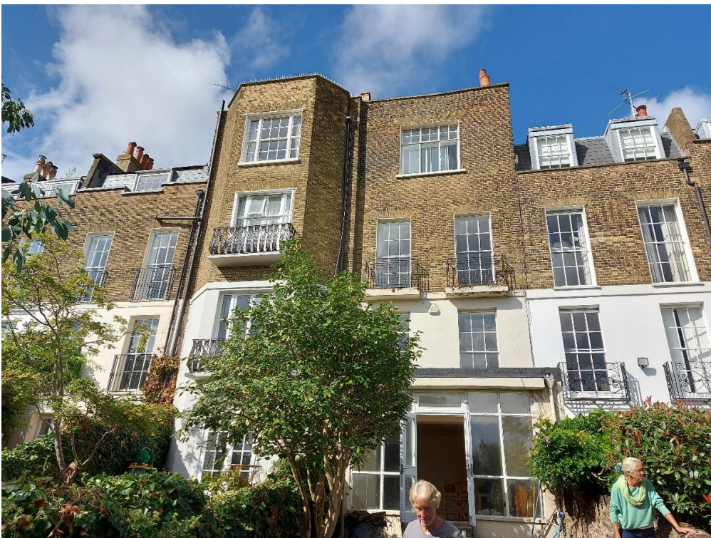
Figure 6: The rear elevation of number 42, to the right of the canted bay of number 40.
