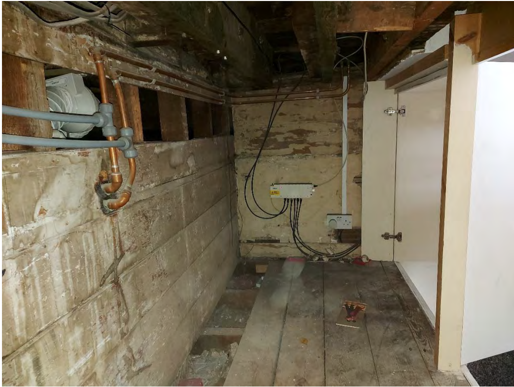
Fig.5: The interior of the cupboard on the stair under what is now the second floor landing, showing the vertical horizontal boarding of what was probably the original stairwell.
