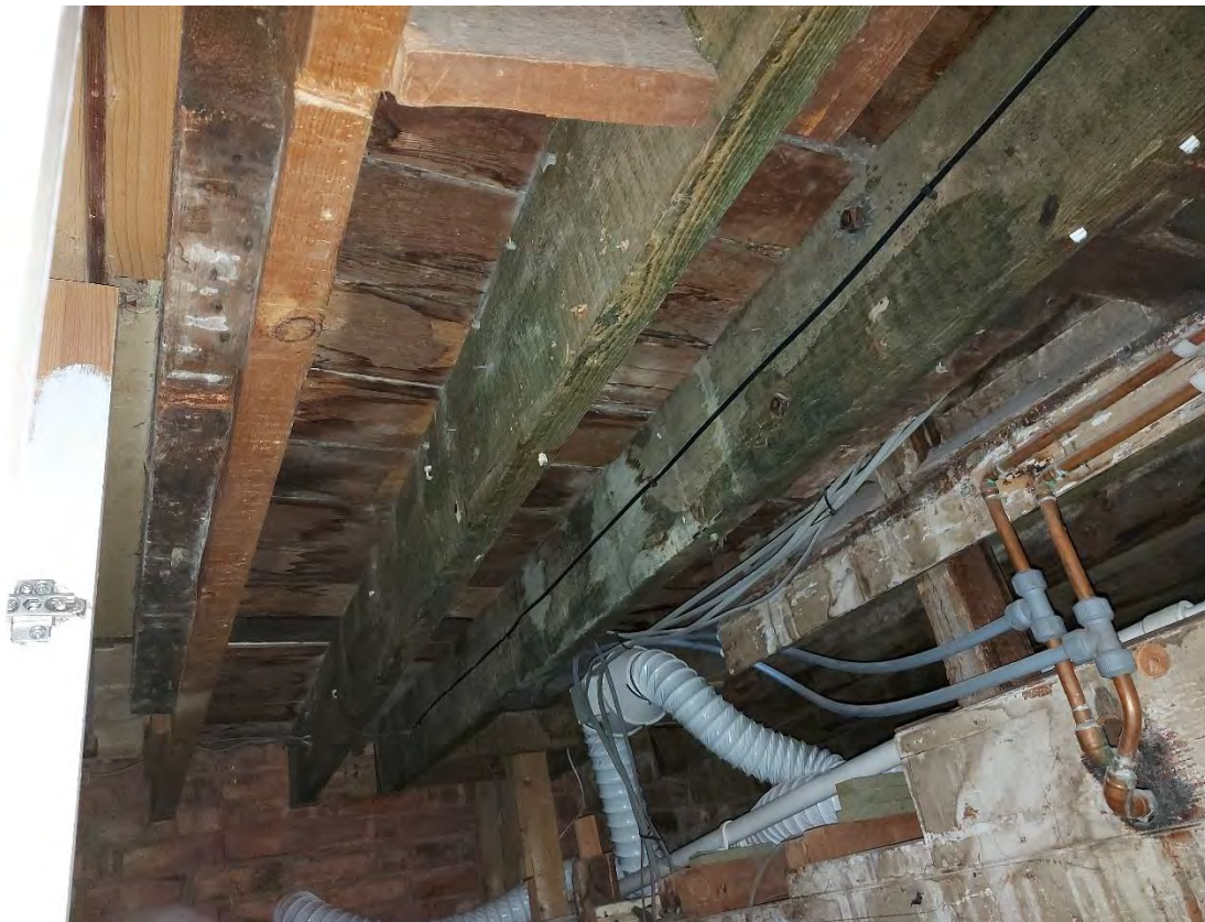
Fig.6: The underside of the second floor landing from the cupboard on the stair, showing the modern joists and also some modern Fletton brickwork in the front wall of the house
