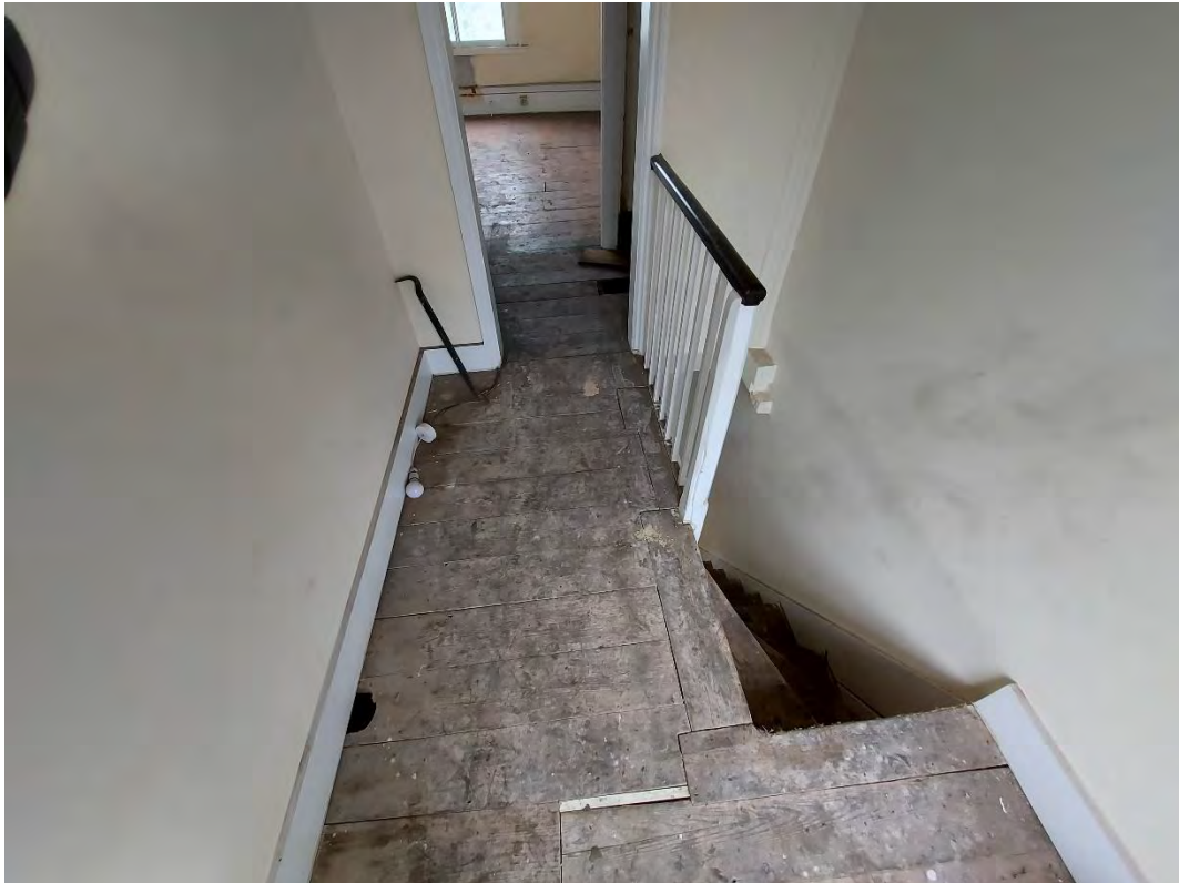
Fig.2: The stair at second floor level
