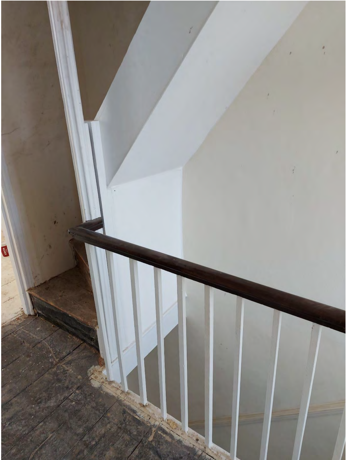
Fig.1: The first floor landing showing the lower part of the upper stair
