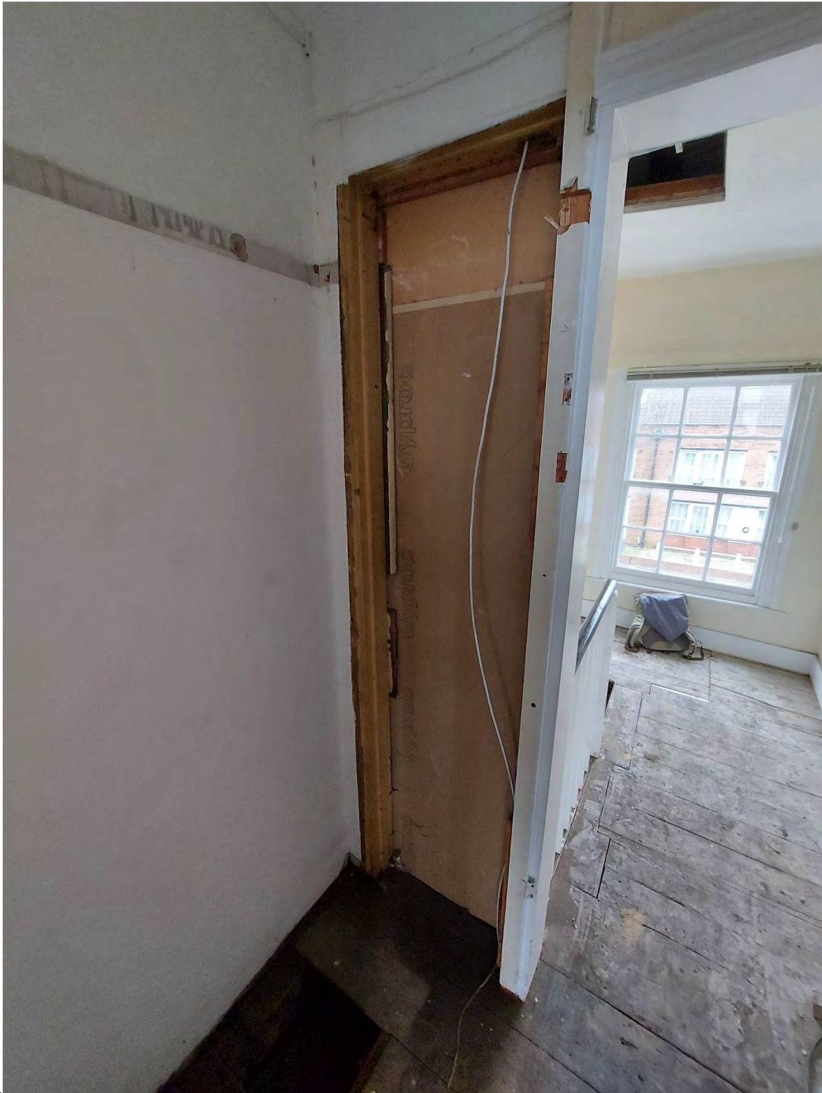
Fig.4: The second floor landing, showing the blocked and truncated former door opening in the lobby to the two main rooms.
