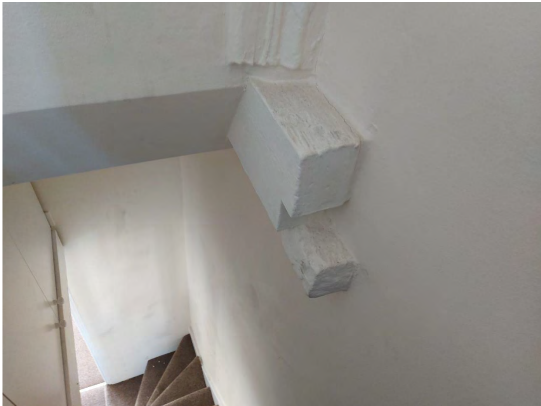
Fig.3: view of the stairwell showing a truncated joist against the party wall resting on a small padstone, and above it the base of the moulded surround to the doorway which now faces onto the stairwell
