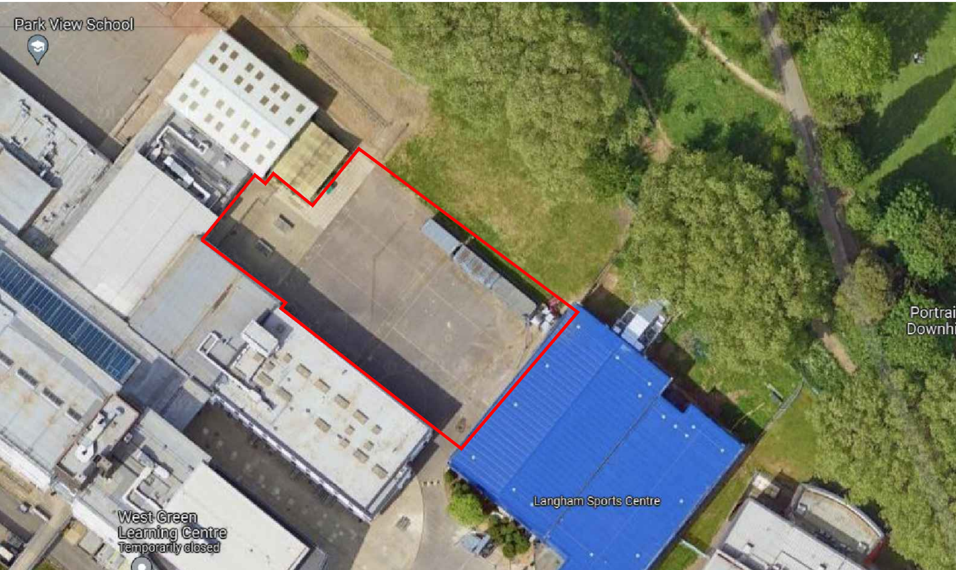
Ariel view As Existing
