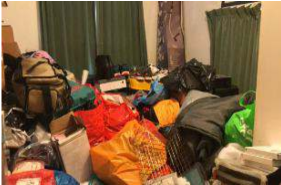
First Floor Rear Bedroom over Outrigger and above Kitchen. Poor access due to Tenants stored items.
