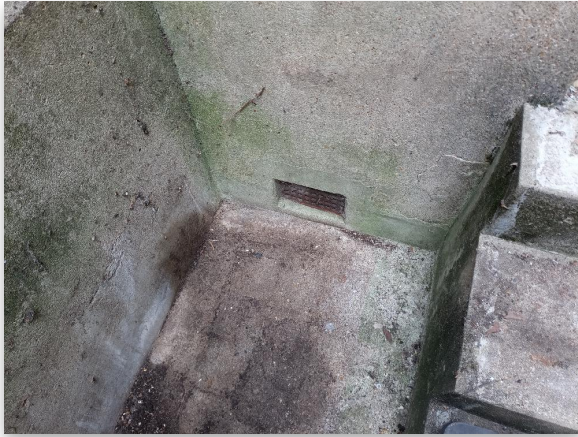
Fig 2.1: Trial Hole 2 Location
