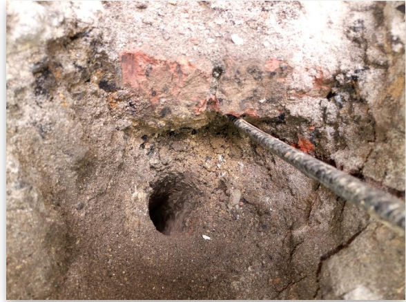
Fig 2.2: Trial Hole 2 Footing
