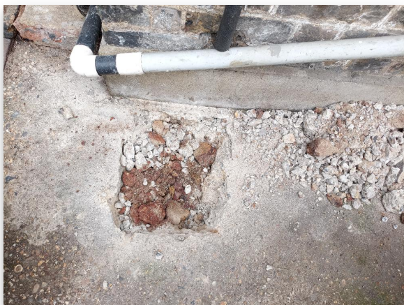
Fig 1.1: Trial Hole 1 Location
