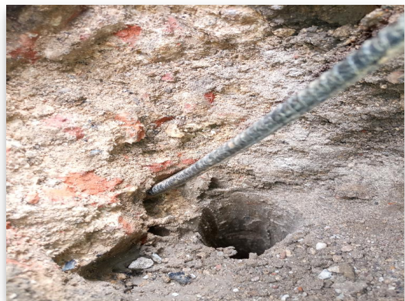
Fig 1.2: Trial Hole 1 Footing
