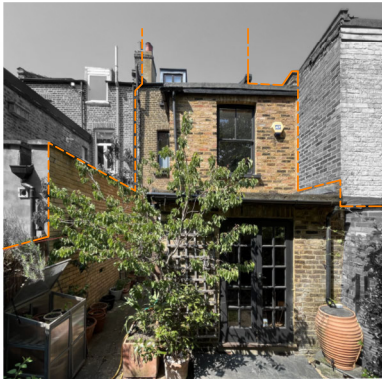
Photo: Garden elevation of 20 Townsend Road
