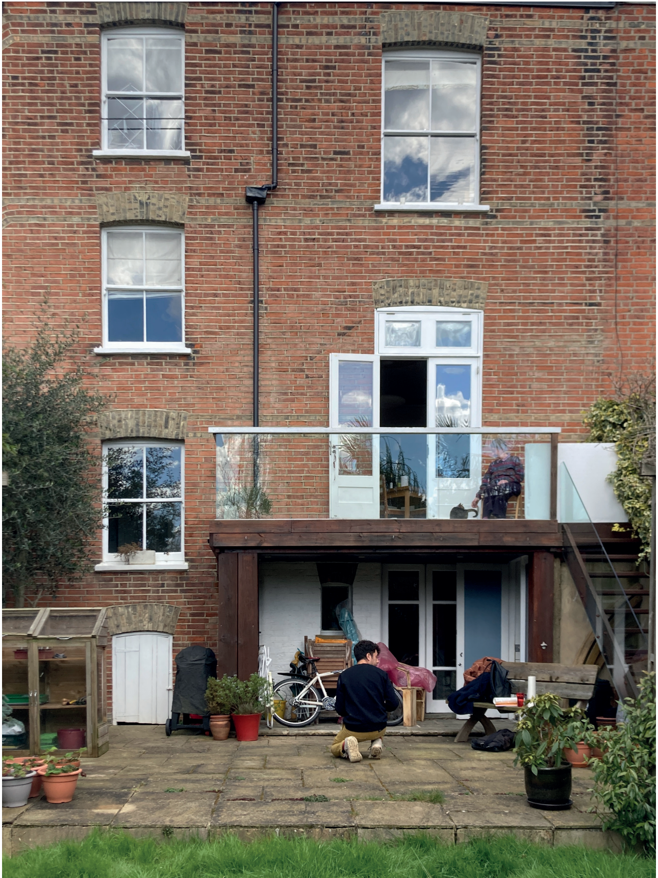
Rear elevation of 98 Stapleton Hall Road
