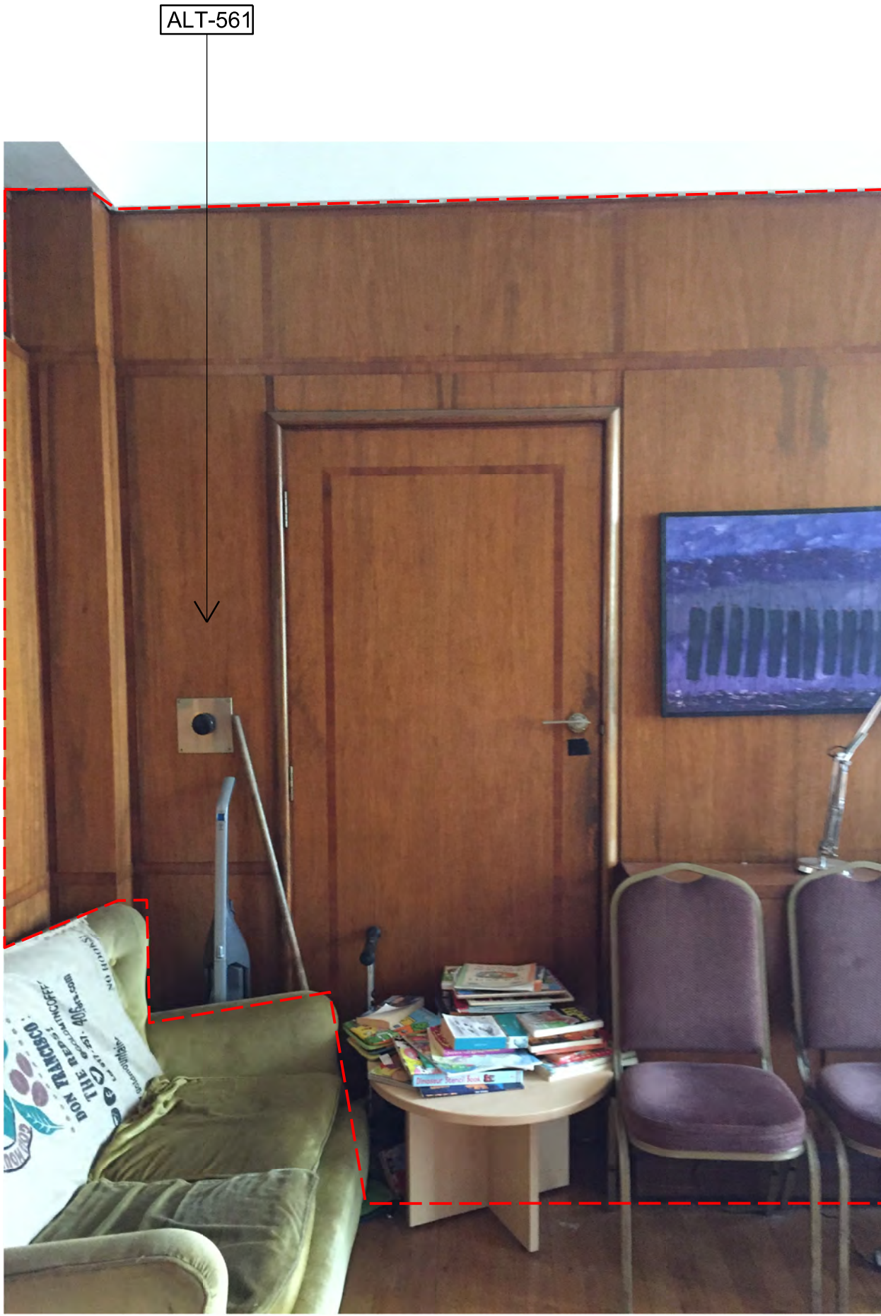
04 Existing timber wall lining 1:NTS
