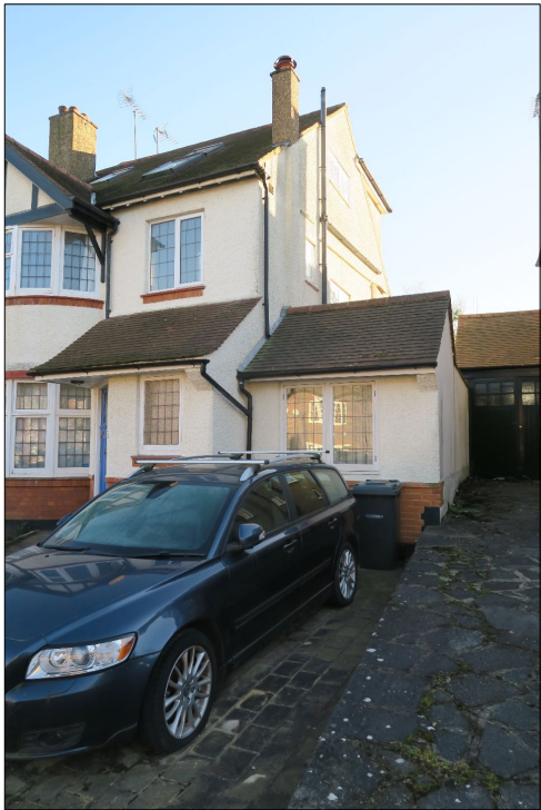
4. front view of side extension at 59 Grosvenor Road
