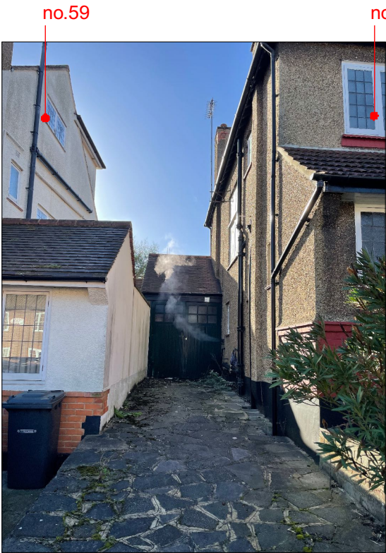
2. view of side alley and existing garage
