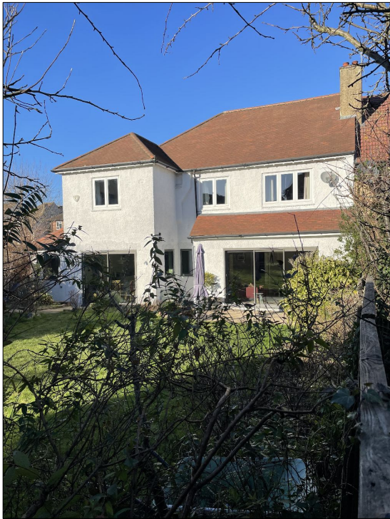
6. rear view of property at 63 Grosvenor Road
