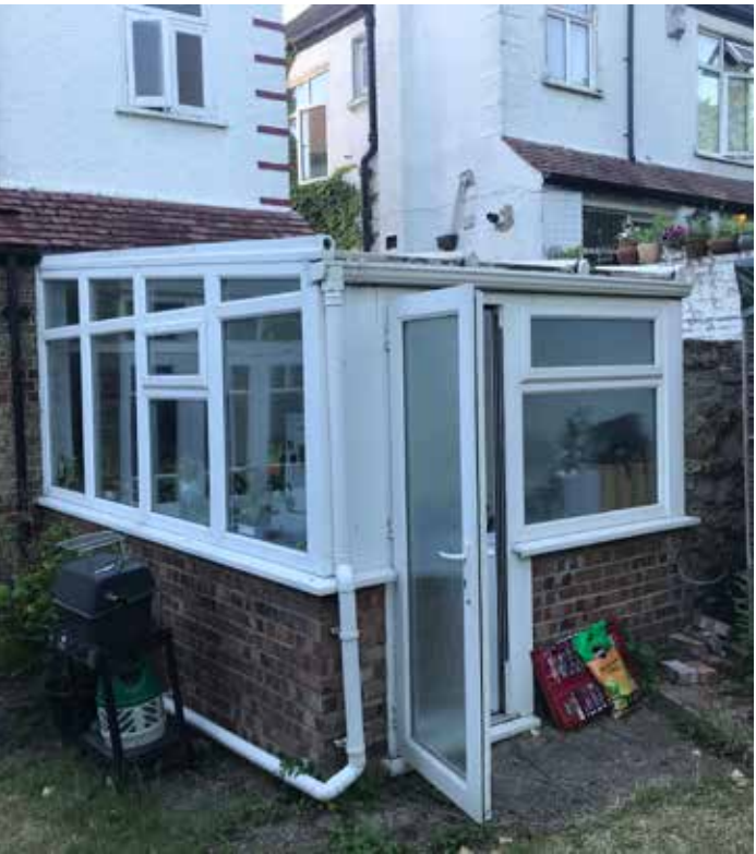
Existing rear extension
