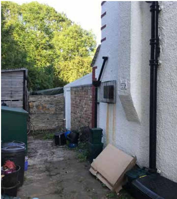
Side passage looking toward the rear
