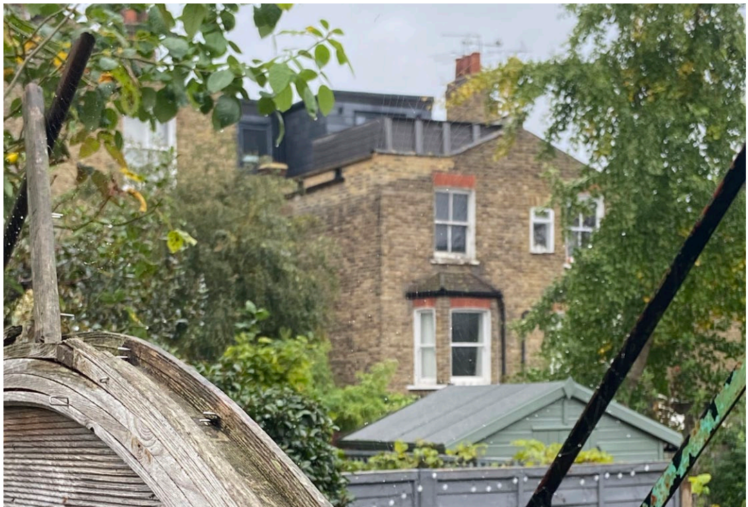
View to double dormer extension and roof terrace at 40 Inderwick Road
