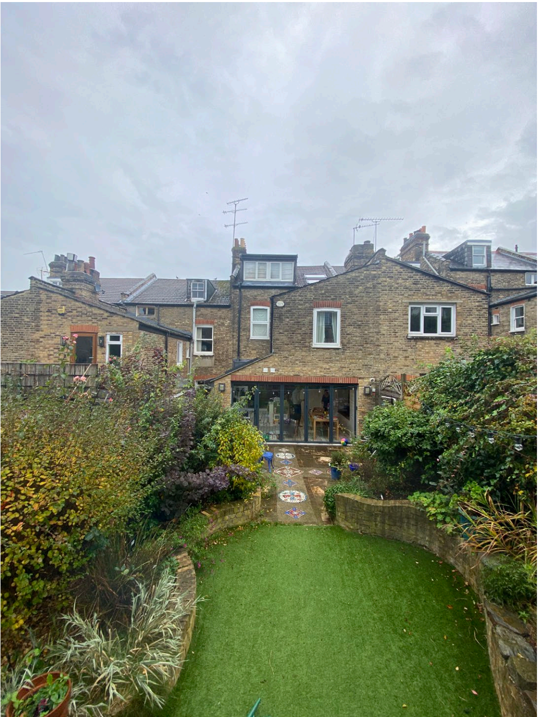
View to rear elevation and 1st floor roof terrace at 37 Mayfield Road
