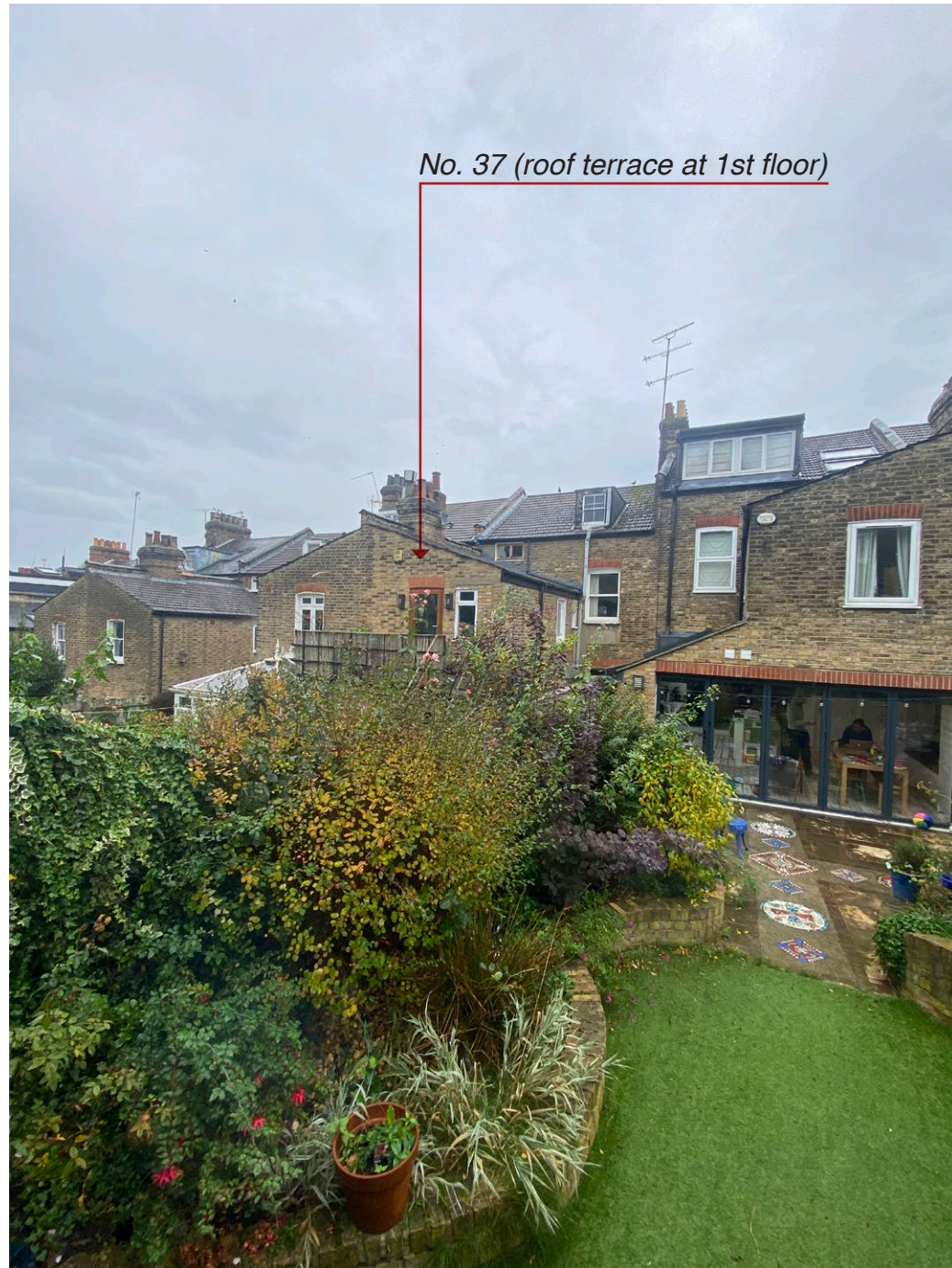
View to 1st floor terrace at 37 Mayfield Road
