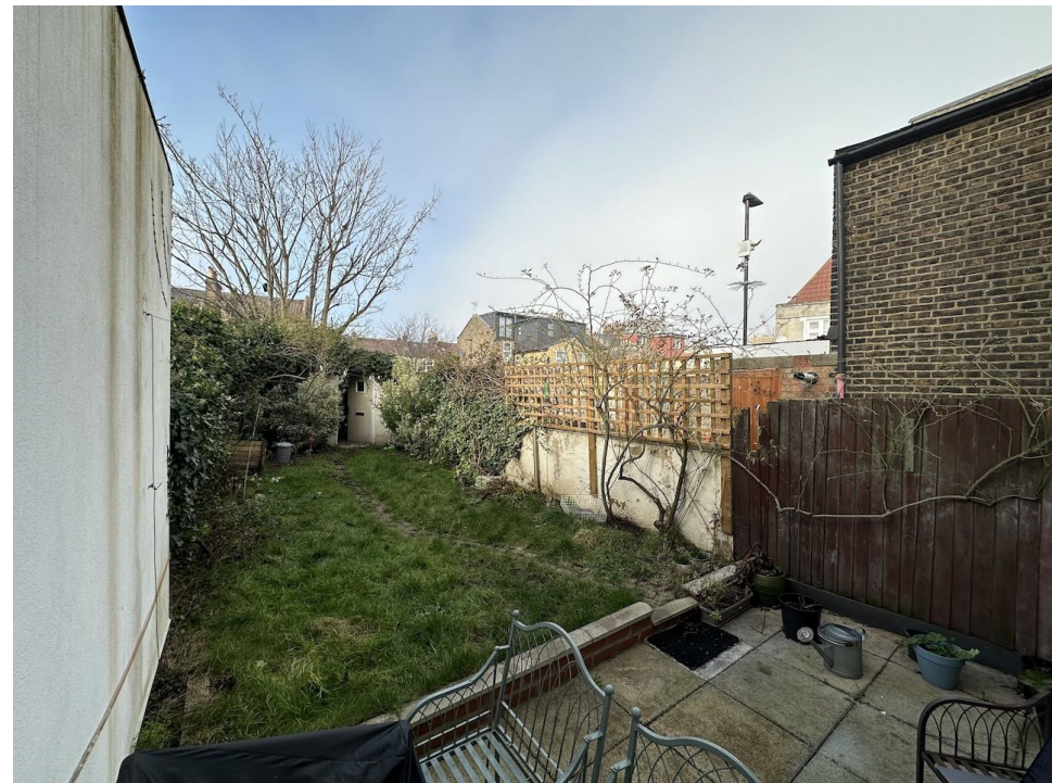
view of N°3 rear garden showing N°5 extension
