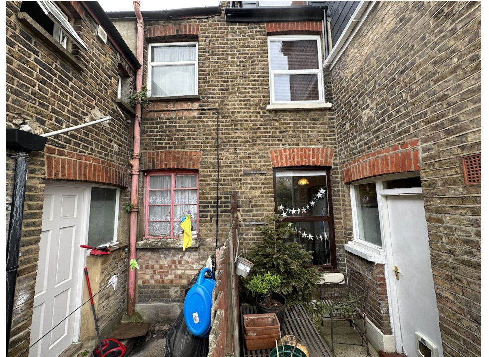
rear view showing relationship between N°1 and N°3
