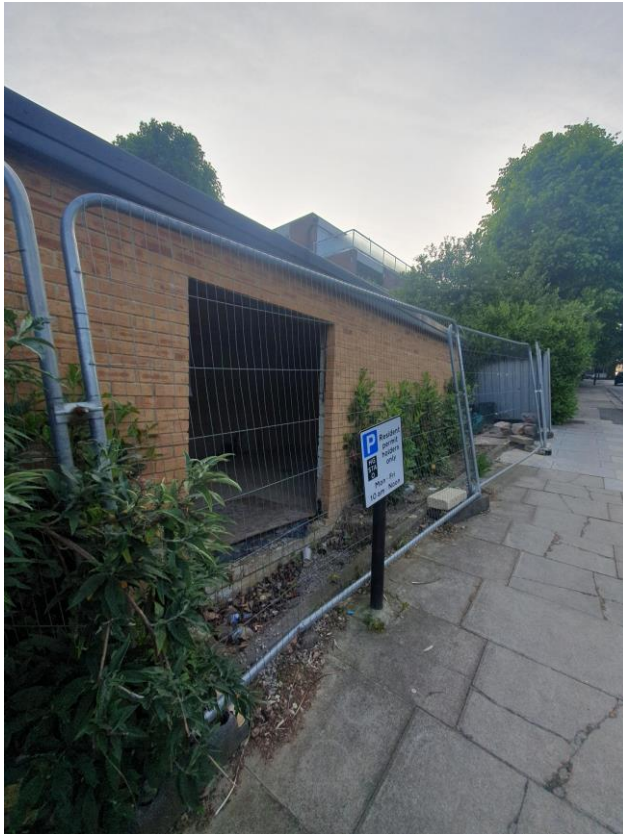
Abandoned bike/bins shed view from the public pavement.
