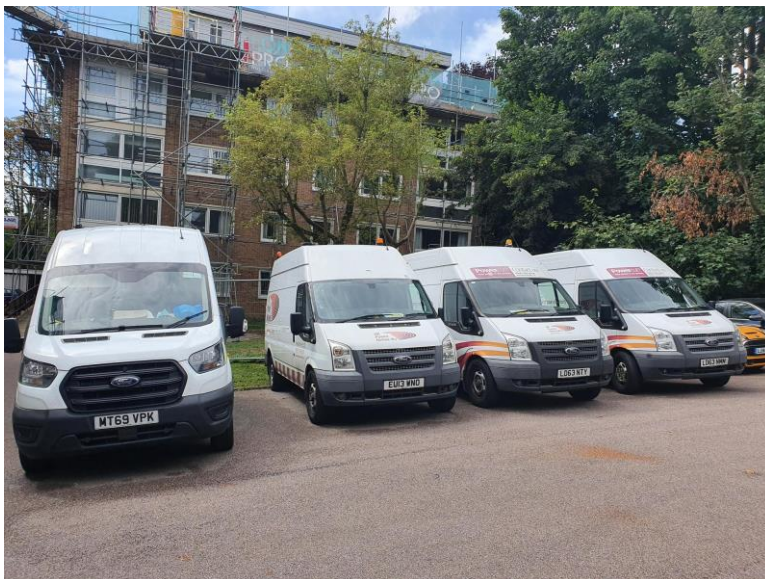
Note the entire front car park being taken over by electricity utility vehicles during electrical works. The contractors said "there is nowhere to park so we're parking in your car park until the work is done."
