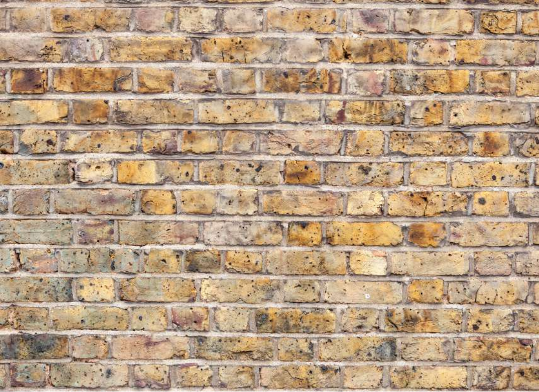
LONDON STOCK BRICK with COAL SPOTTING
