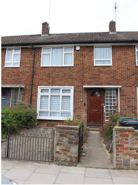
Front Elevation Photo taken 06.06.2023
