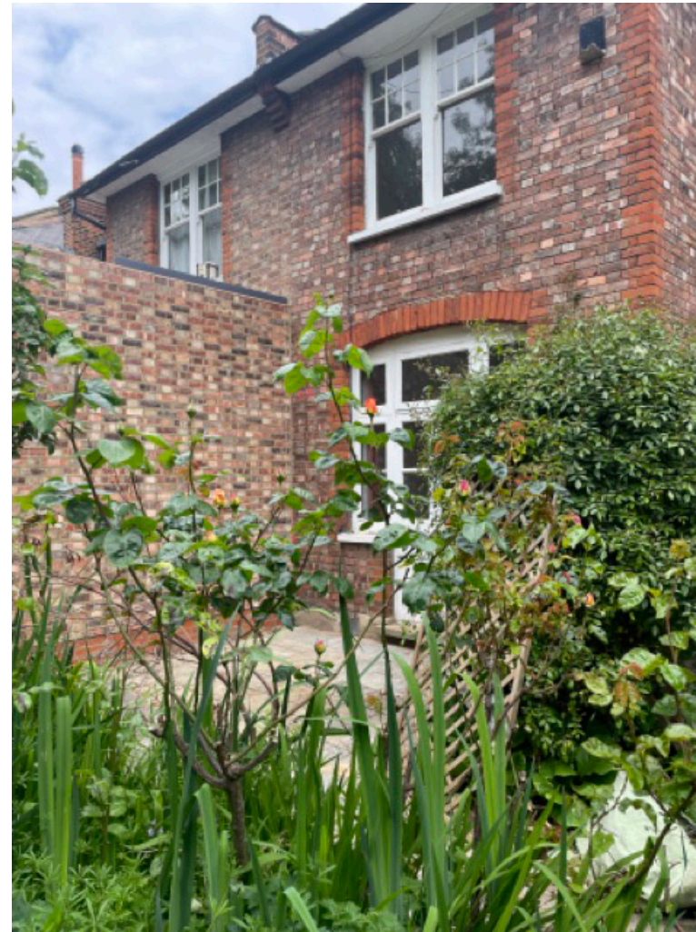
Neighbours Extension and area to be lowered to achieve internal height.
