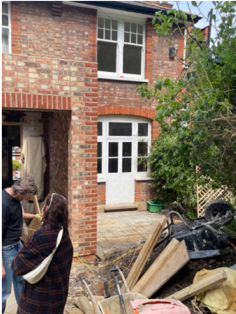
Looking at 32 Glassylyn Road rear elevation from neighbours extension
