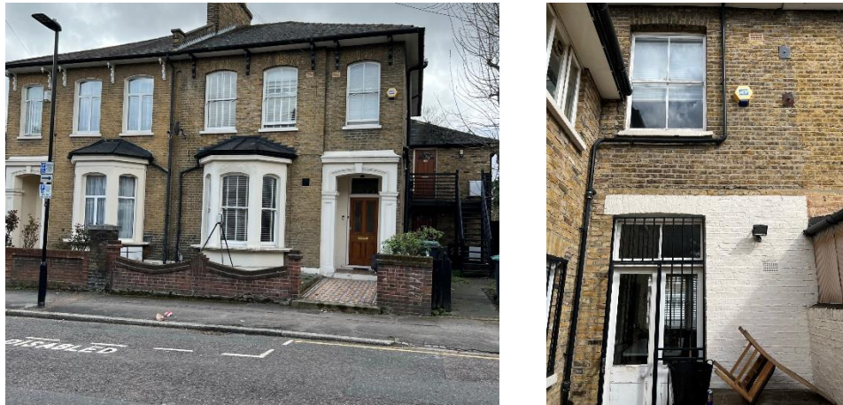
Figure 2: Existing windows on front and rear elevation
