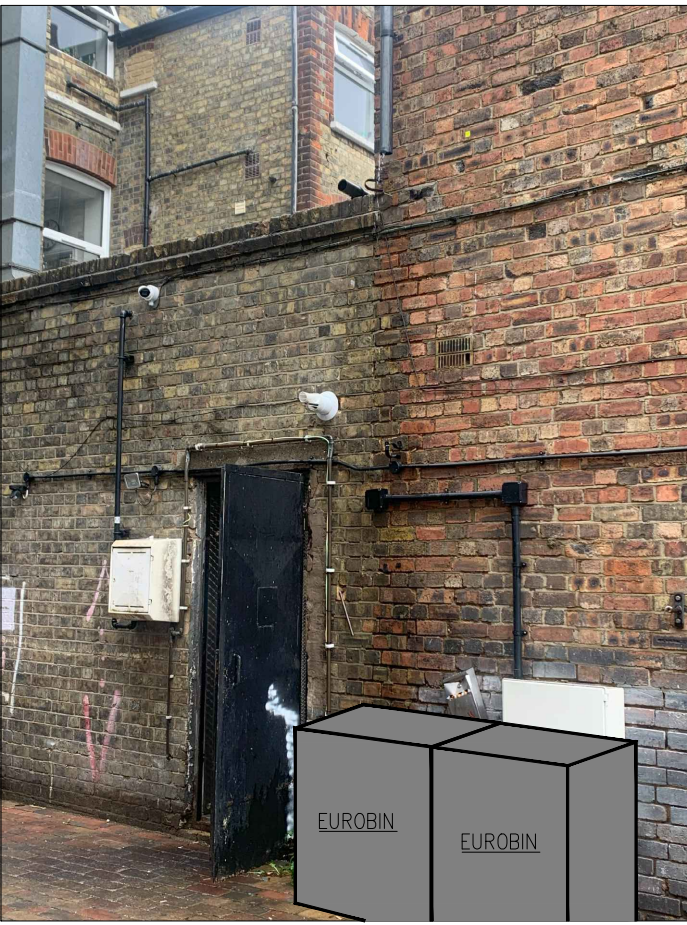
IMAGE 1 – EXISTING HARD STANDING AREA IN ALLEYWAY
