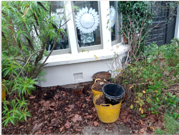
Fig 1.1: Trial Hole 1 Location
