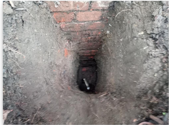
Fig 1.2: Trial Hole 1 Footing
