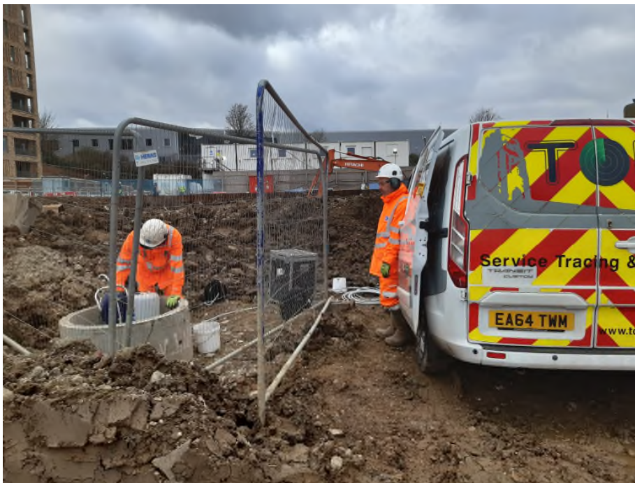
Plate 2: Site attendance by TOR drilling on 22 nd February 2022 to decommission BH514A. 270-300l of bentonite grout (50kg of grout per 70l of water) was pumped into the standpipe via tremie pipe.
