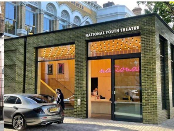
Contemporary glazed brick extension to a Victorian building in Islington
