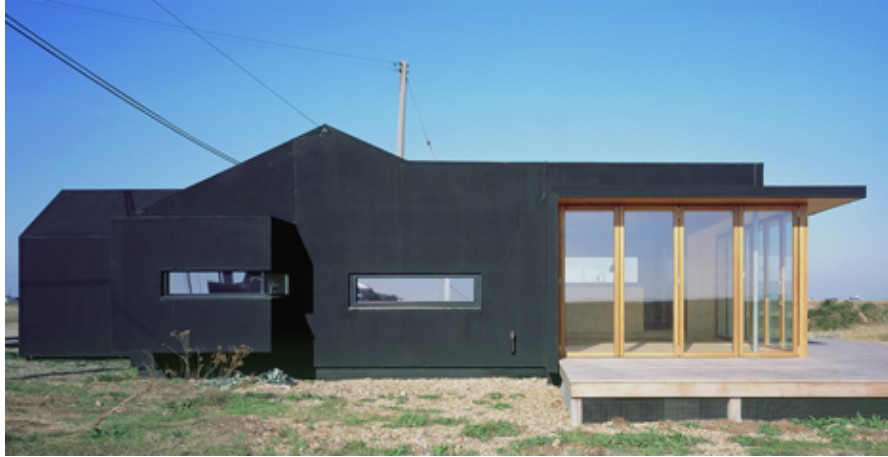
Black Rubber Beach House by Simon Conder Associates
