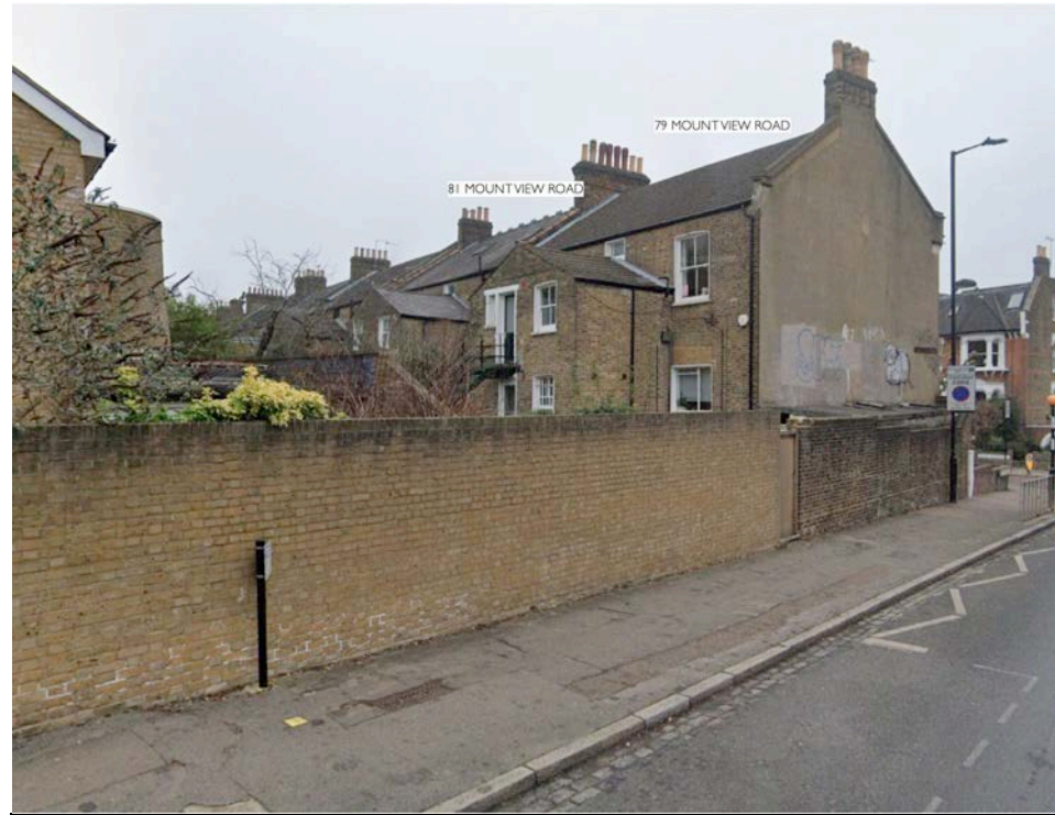
View of 81 Mount View Road from Ferme Park Road
