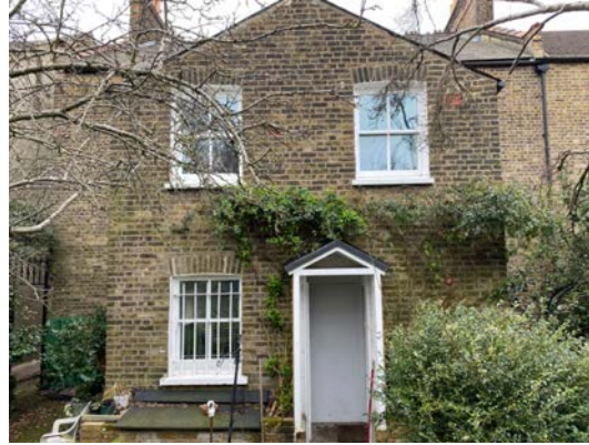
Rear elevation of existing house showing double pitched roofs
