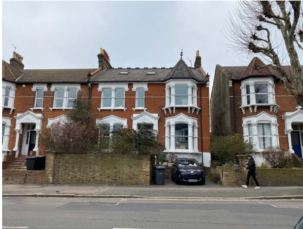
Photograph of front elevation showing existing roof lights
