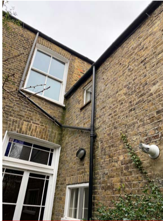
Existing window in side elevation of first floor of outrigger
