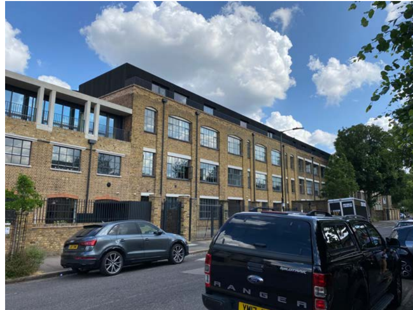
EPDM Roof Extension on a Victorian Building in De Beauvoir Town Hackney
