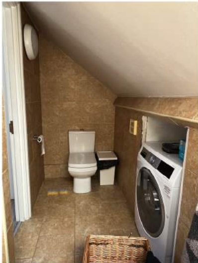
View of existing ensuite at second floor
