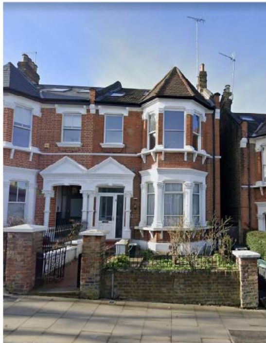
View of the street-facing elevation
