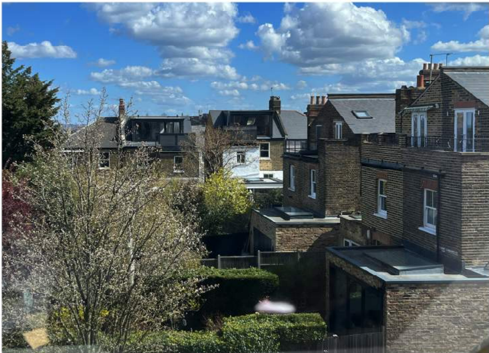
View looking out from the front (East) of the property from second floor demonstrating consented roof terraces at Dashwood Road and Ferme Park Road
