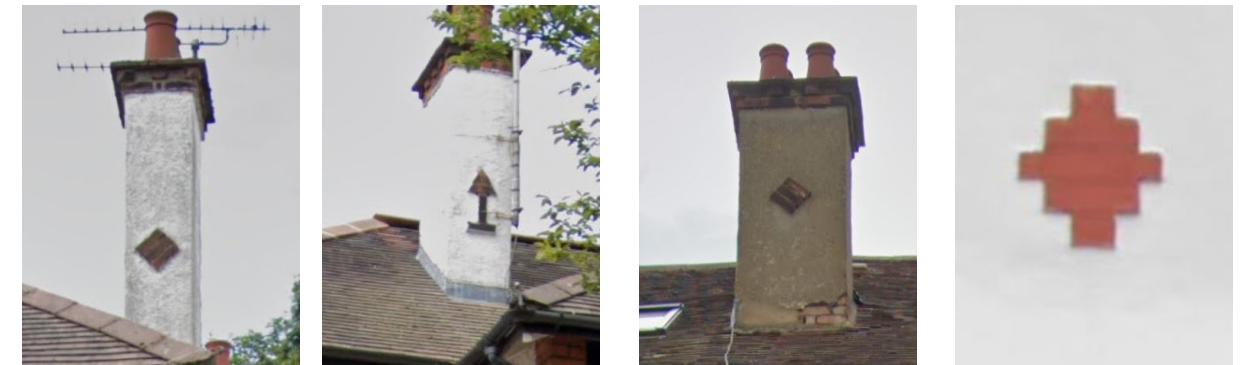
Brick detailing of chimneys along Cholmeley Crescent
