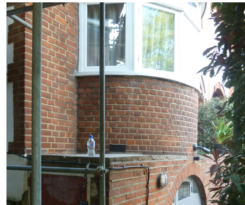
Front Elevation of No. 45 showing semi-circular brick bay window
