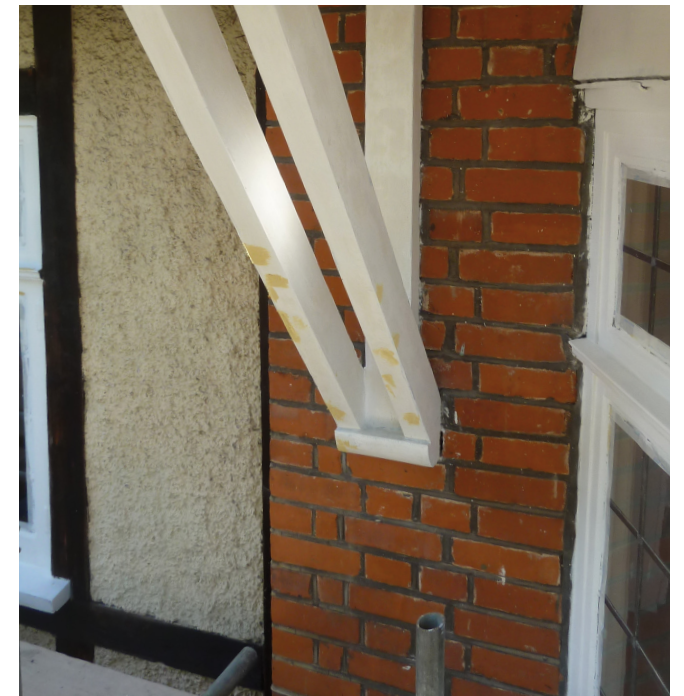
Rough render, brickwork and painted timber of No. 43
