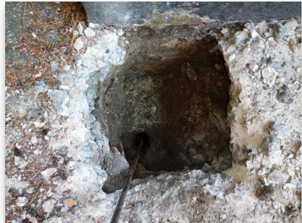
Fig 1.2: Trial Hole 1 Footing
