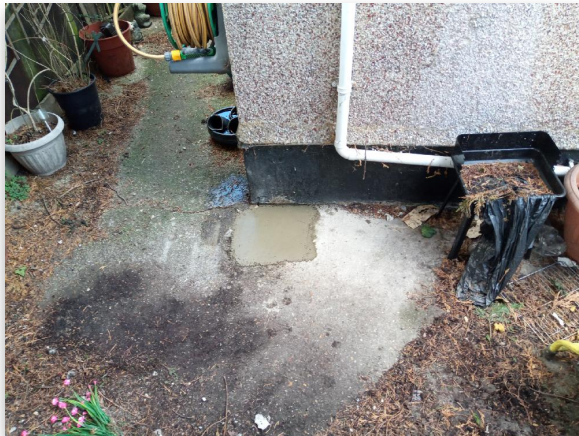
Fig 1.1: Trial Hole 1 Location
