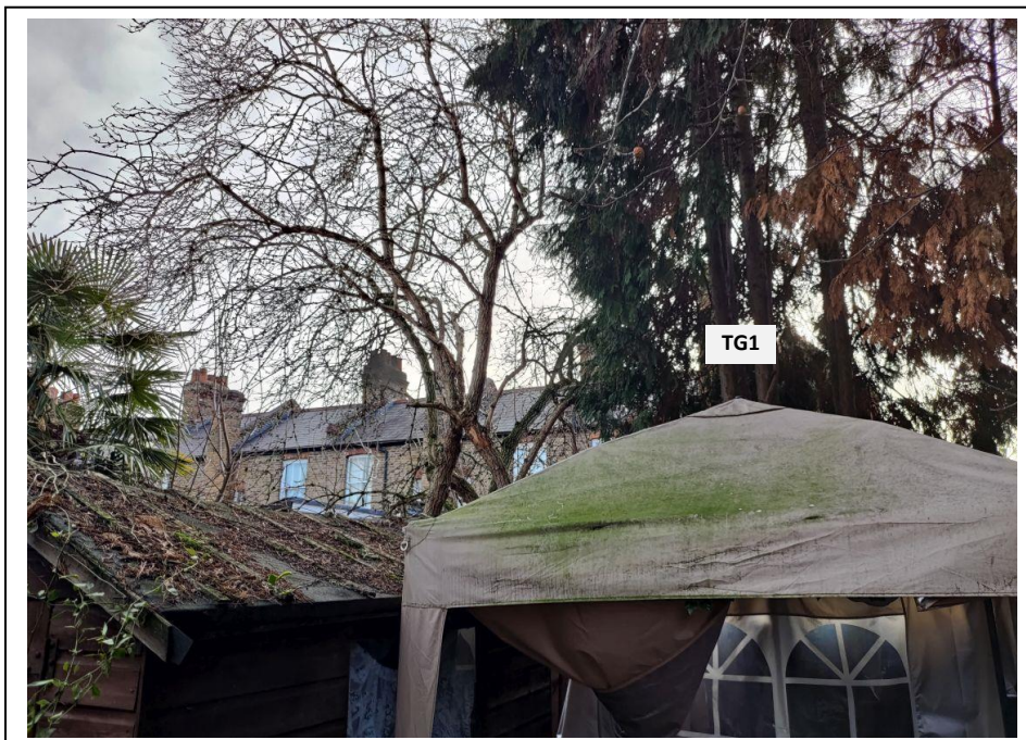
View of rear boundary elements of TG1 group
