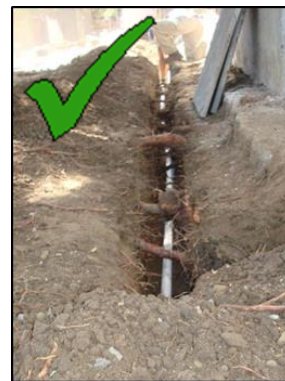
Significant roots retained.
