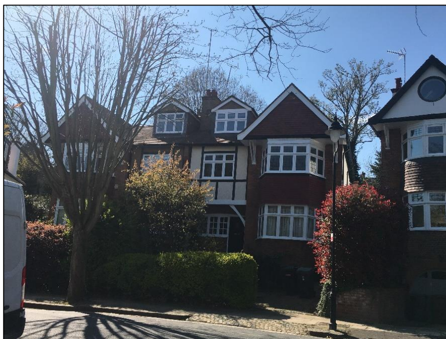
Photo 3: View from front – Ash T10 and Sycamore T1 visible to rear (smaller trees obscured by property with minimal visual amenity value).
