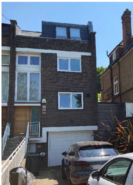
Figure 1: Photograph of the property as viewed from the public high street of Woodview Avenue
