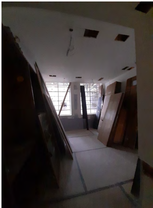
109B F.21 Hotel Room (Former Medical Officer's Room)
