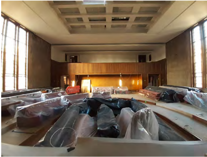
112 F.33 Council Chamber looking north to Public Gallery
