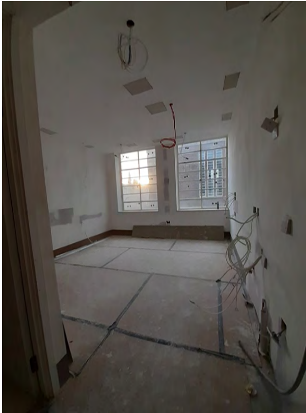
109D F.21b Hotel Room
