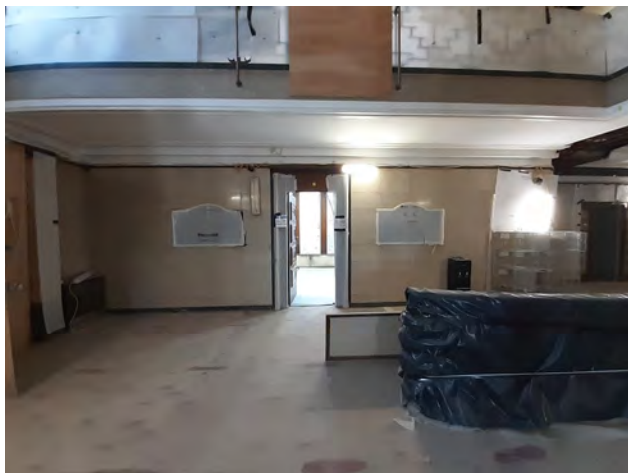
119 F.44 First floor landing arriving at the top of stairs, looking east
