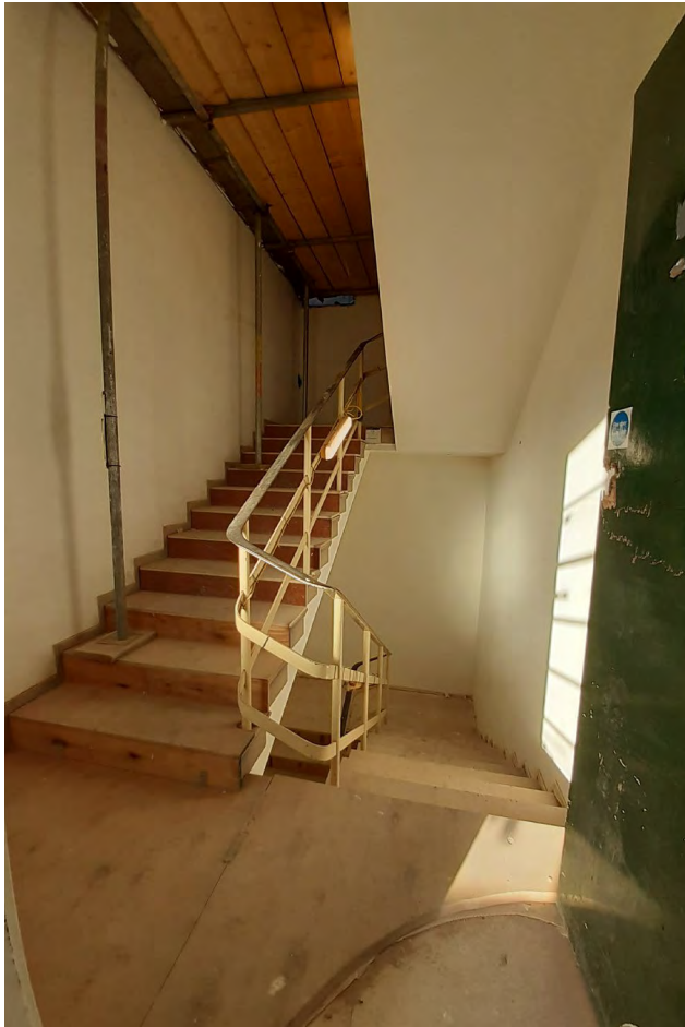
152A ST.04 first floor (stair closed off at second floor)
