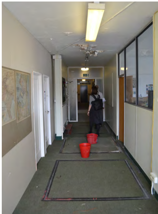
110A First Floor, corridor in east office wing, F.28 (2017)
