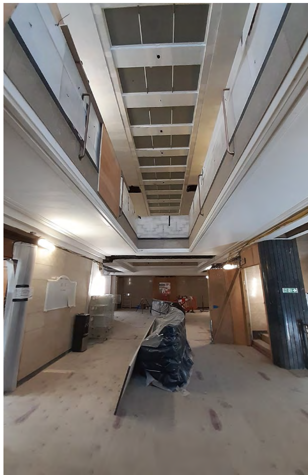
119A F.44 First floor landing, looking south to Council Chamber
