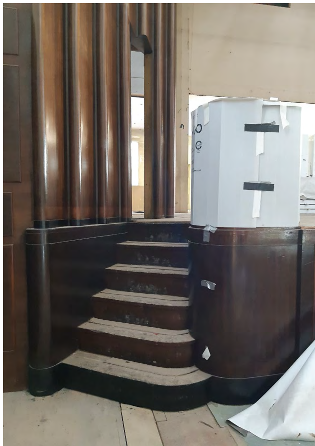
95C G.57 Assembly Hall, showing timber stairs up to stage and part of proscenium
