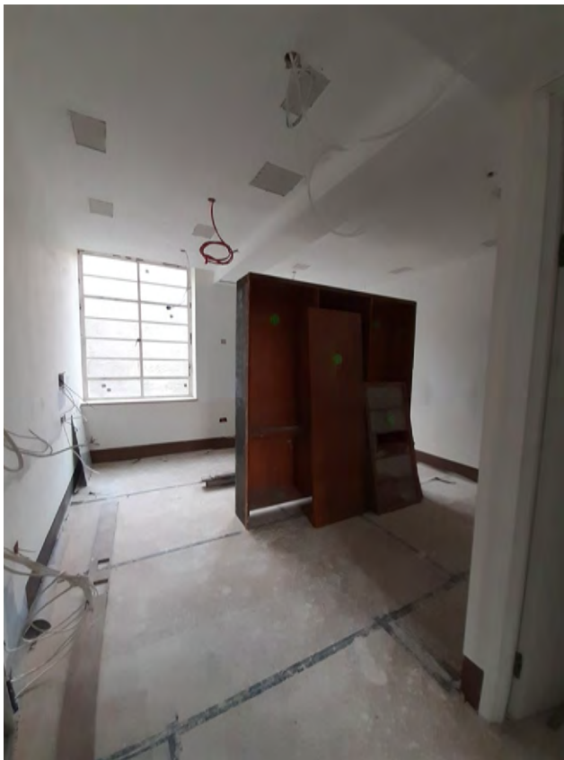
104A F.6 Hotel Room Former Deputy Town Clerk's Room
