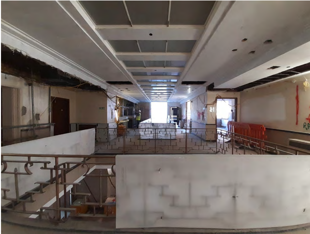
142A S.33 Second floor landing with S.32 in foreground and S.34 in background
