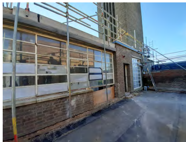
130A S.1a Roof Terrace looking west to Tower
