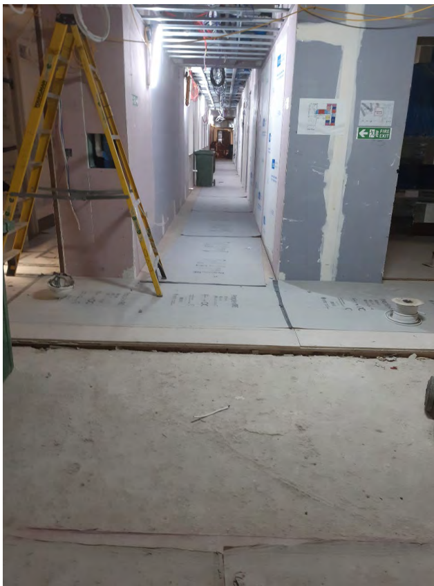
110 F.28 Corridor looking south
