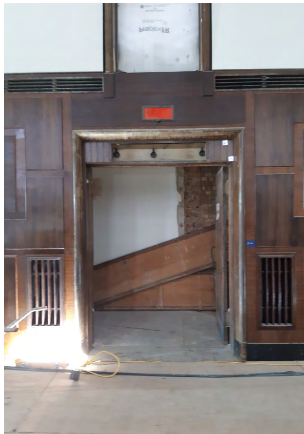
95D G.57 Assembly Hall panelled fire exit doors
