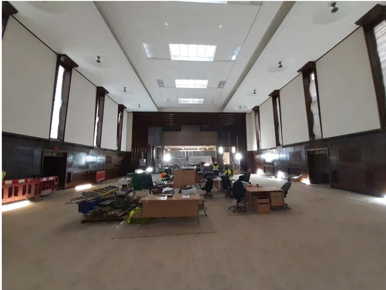
95 G.57 Assembly Hall looking to east (stage)
