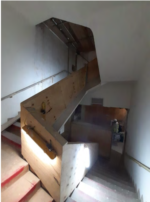
150 ST.01 view at ground floor
