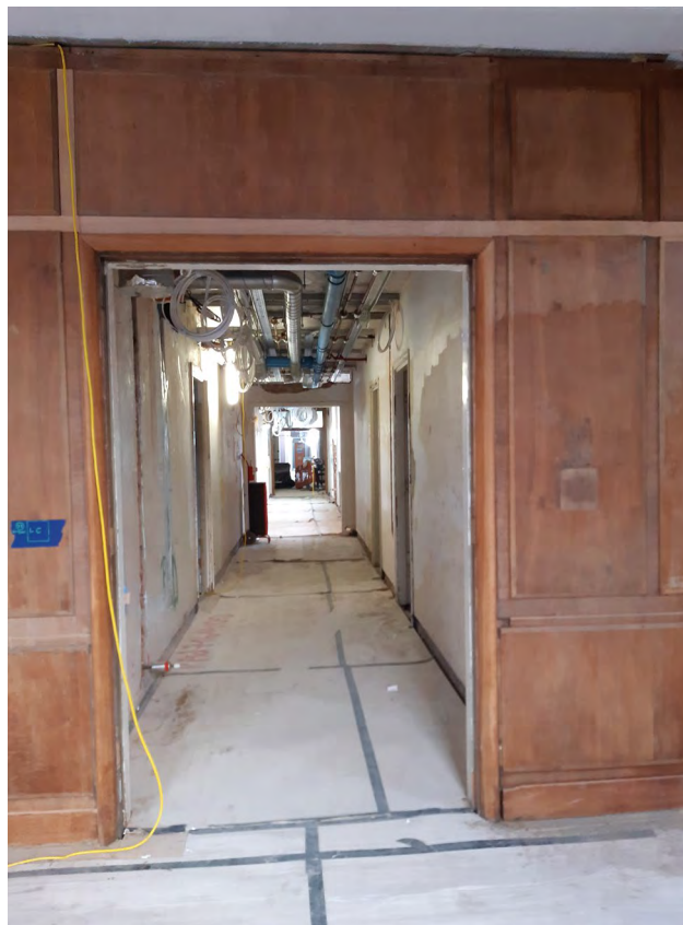
113A F.36 Lobby viewed from F37 Member's Room
