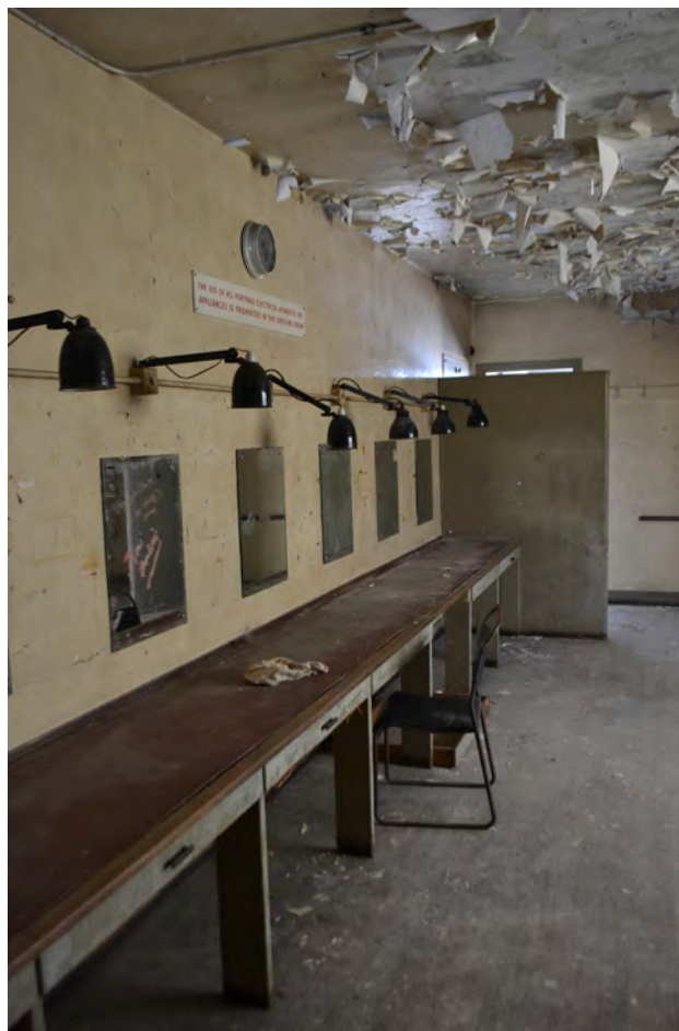
123A First Floor, former ladies' dressing room, F.51 (2017)
