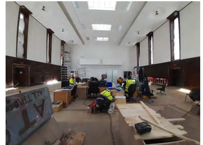
95B G.57 Assembly Hall looking west to Function Room and Foyer
