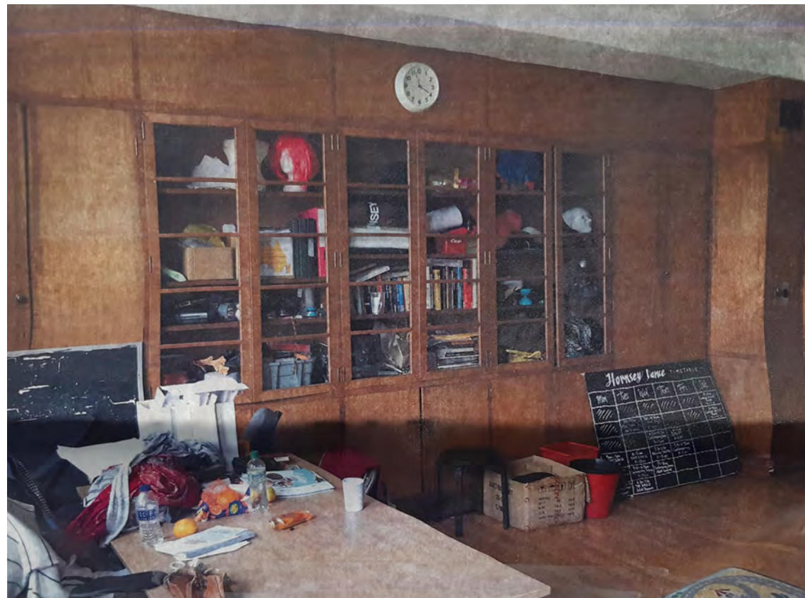
76B G.15 Hotel Room original cabinetry to be rebuilt in room (historic image in room)
