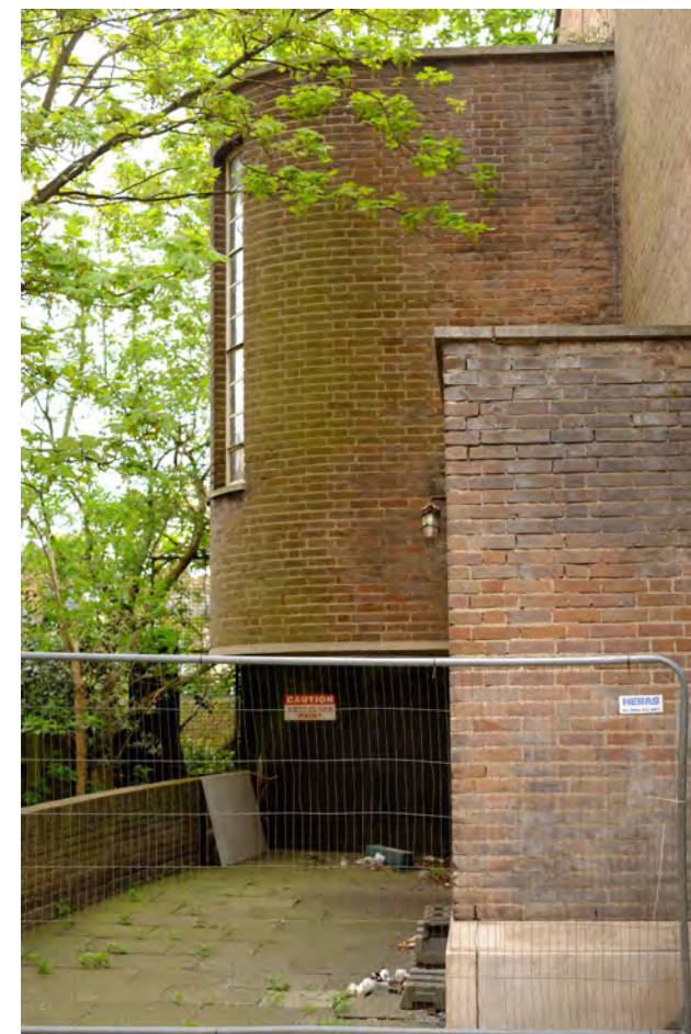
34 North elevation of the Assembly Hall Block, cantilevered stair (2017)
