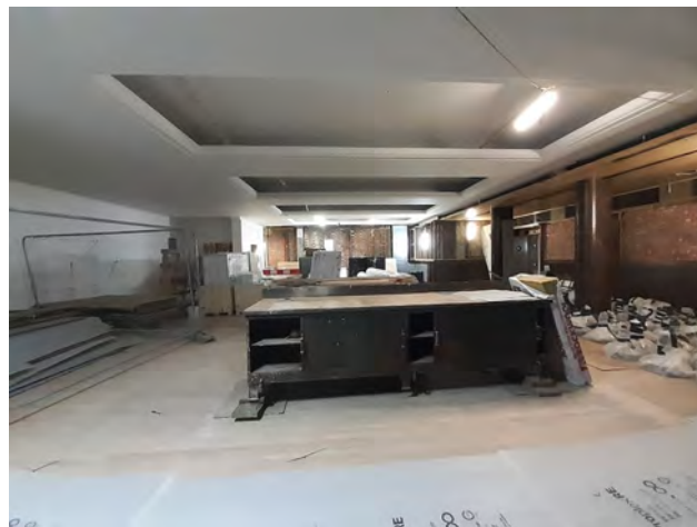
94A G.55a Function Room looking south; image shows some retained furniture and lighting fixtures being stored for re-use
