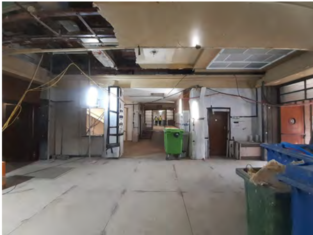
93A G.55 Foyer looking towards G.41 Entrance Hall
