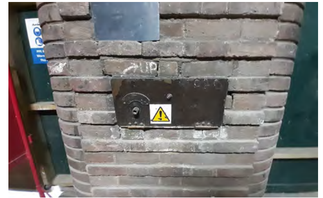
89D G.49 Vestibule switchplates and fittings set into decorative brickwork
