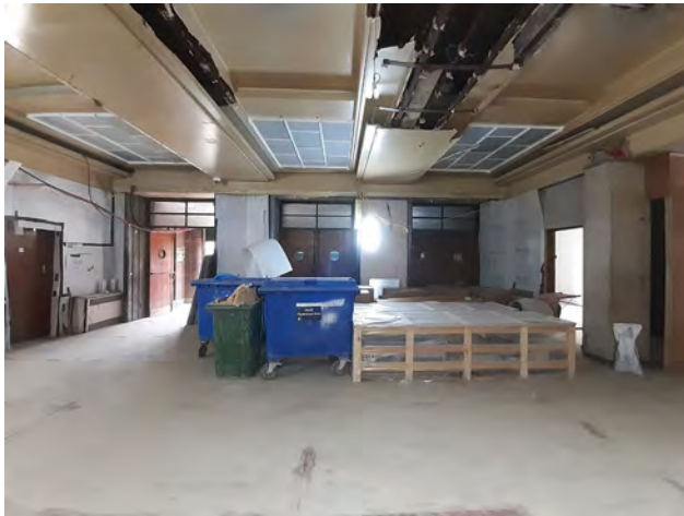
93 G.55 Foyer looking towards Assembly Hall
