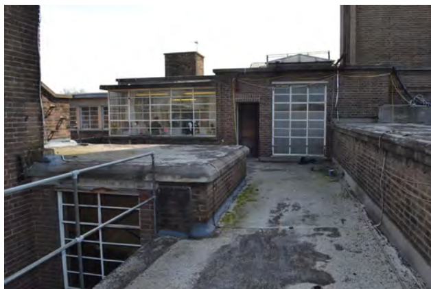
44 Flat asphalted roof over Assembly Hall Block (2017)
