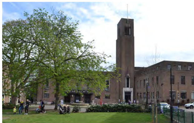
30 Main elevations of Hornsey Town Hall (2017)
