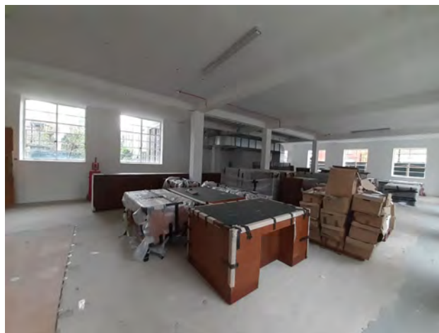
81A G.38 F&B Restaurant Cafe looking southwest to kitchen prep area (by others)
