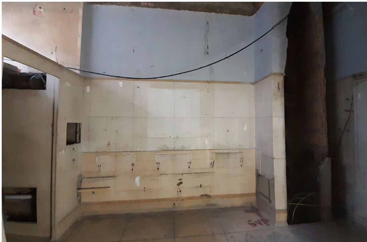
87A G.45 Men's Lavatory looking south
