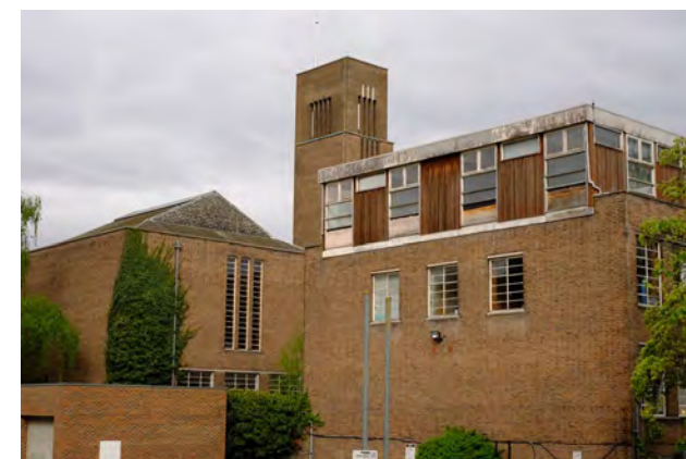
39 South Elevations (2017). Note that timber extension to right now replaced with a new storey providing hotel accommodation to the second.
