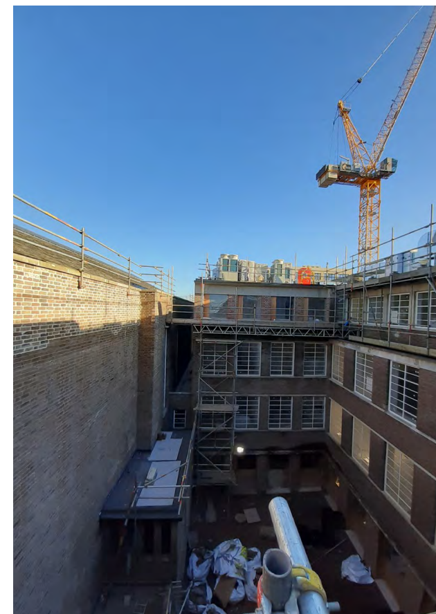
43 Hotel courtyard elevation looking east
