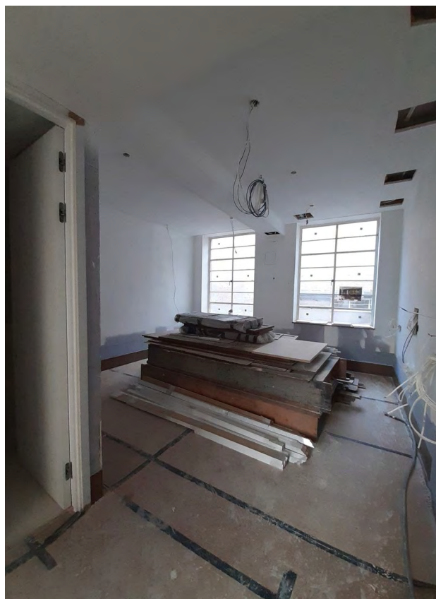
73 G.8 Hotel Room Former Borough Treasurer Room (furniture for reassembly)
