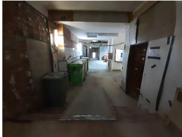
93D G.46 Corridor looking towards G.55 Foyer
