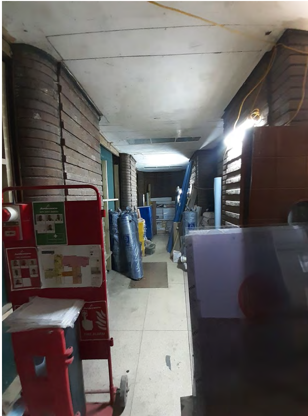
89 G.49 Vestibule looking north
