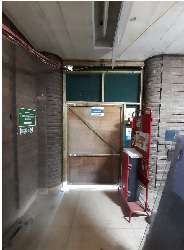
89A G.49 Vestibule, entrance door opening
