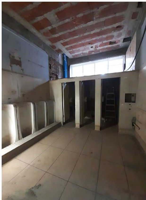
87 G.45 Men's Lavatory looking east
