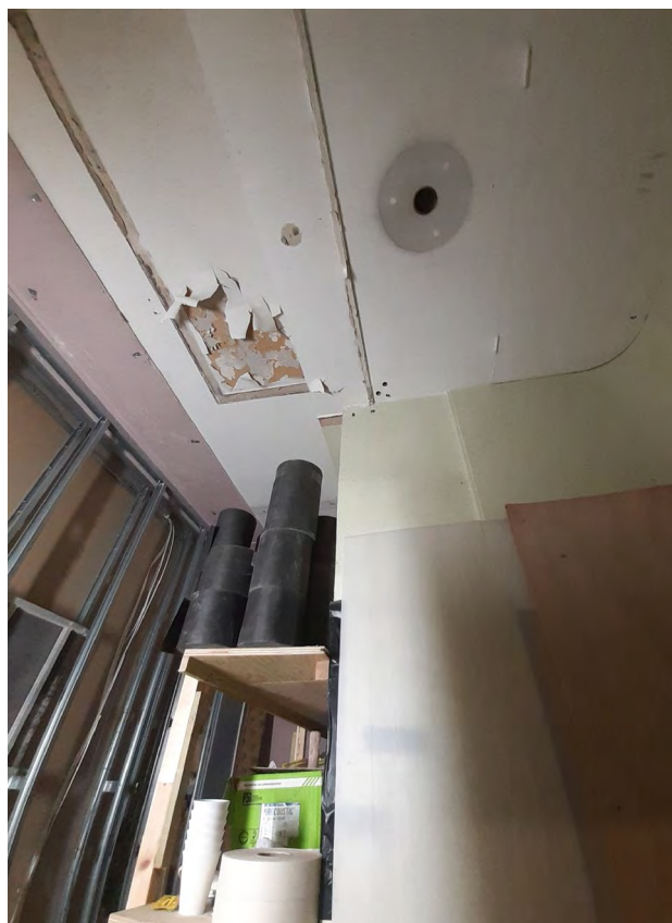
70 G.2 Concierge interior showing curved wall and painted ceiling
