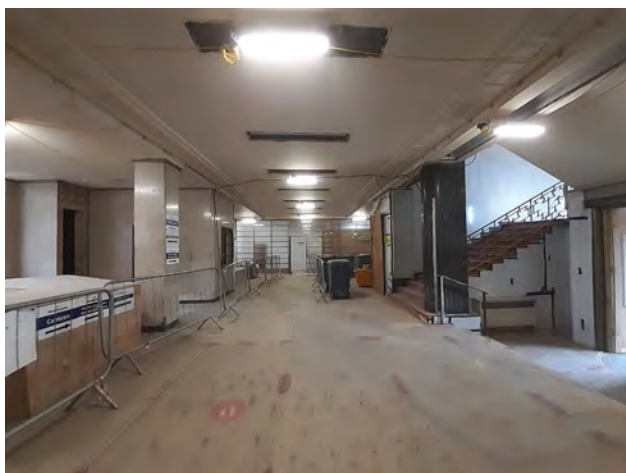
85A G.41 Entrance Hall looking south, with the main entrance on the right
