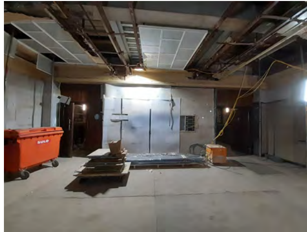
93B G.55 Foyer looking towards Assembly Hall
