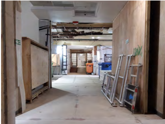
93C G.52 Corridor looking towards G.55 Foyer
