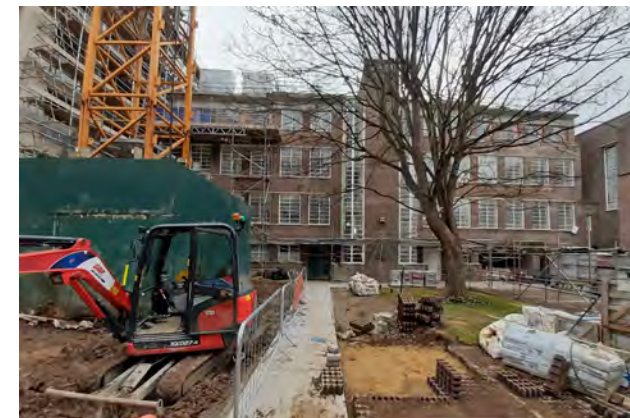
36 Rear (east) elevation of the east office wing, second floor extended to length of east office wing
