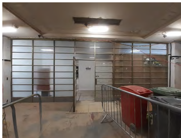
85D G.41 Entrance Hall screen at south end
