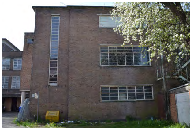
35 Rear (east) elevation of Assembly Hall Block (2017)
