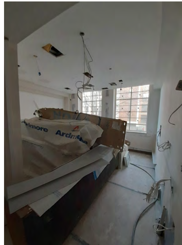
79B G.19b Hotel Room (original furniture for reassembly in room)
