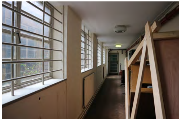
53C LG.20 Basement, corridor in Link Block (2017)
