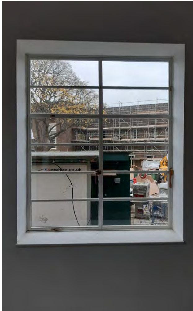
81C G.38 F&B Restaurant windows (original)
