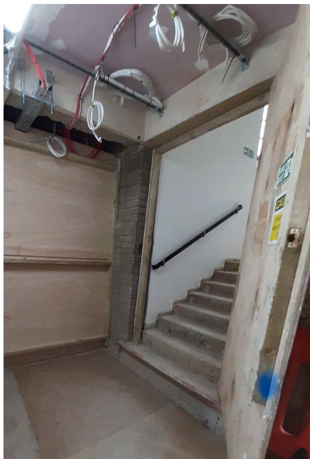
50A LG.03 Entrance Hall Basement
