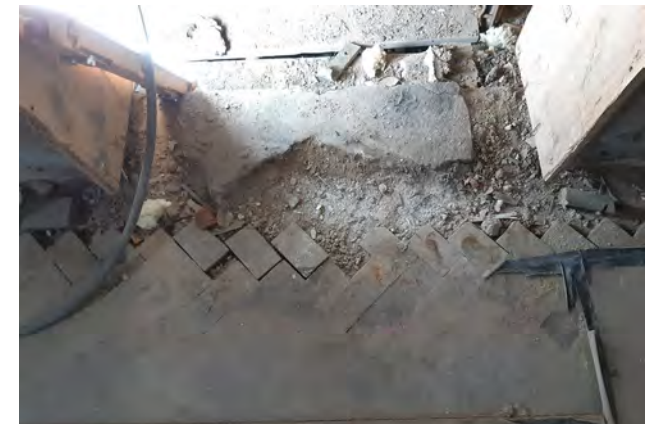
59B LG.28b Corridor floor showing original parquet floor blocks
