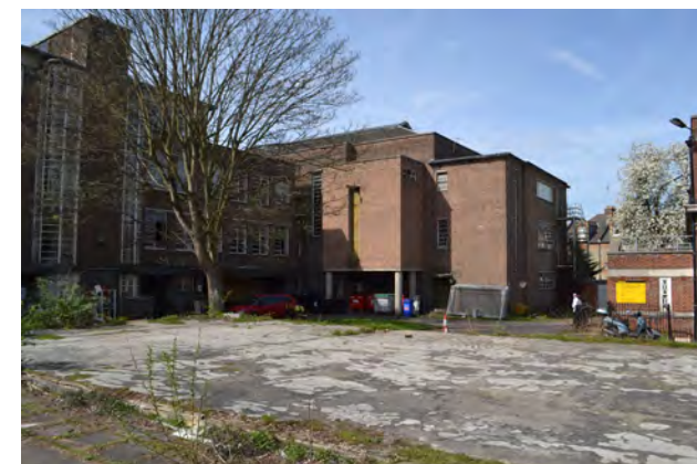
38 South elevation of Assembly Hall Block (2017)
