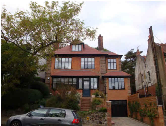
Black steel windows close to face of brickwork and other significant changes permitted
