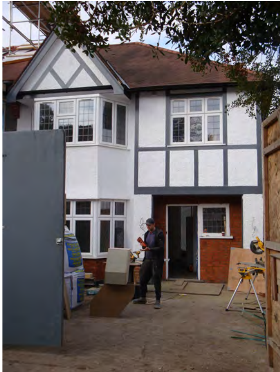
Careful restoration in same group as no. 18
