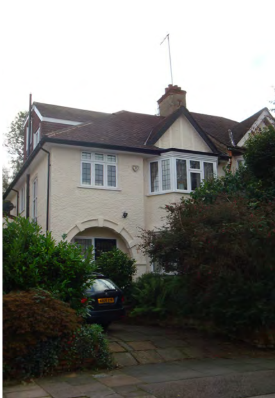
Inappropriate side dormer - not recent
