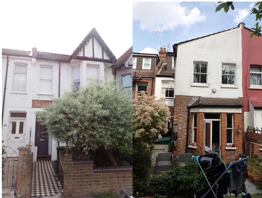
23 Bourne Road Front elevation
