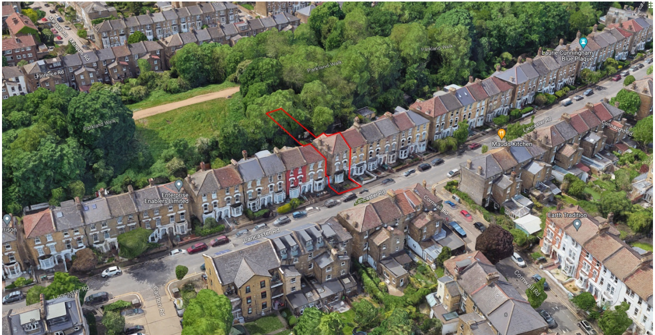
Aerial View of Site
