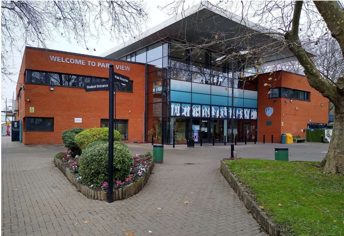
PARK VIEW SCHOOL TEMPORARY MODULAR CLASSROOMS
