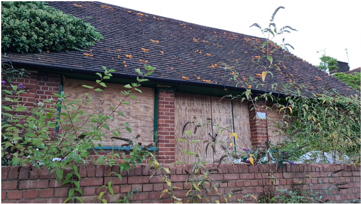
Plate 1 External view of The Pavilion (foam can be seen across the roof line)
