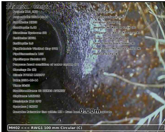
20211014-093650-snap0000.jpg, 00:00:00, 0.00 m Start node, manhole, reference: MH02
