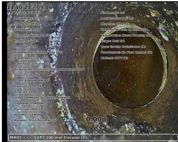
20211014-091654-snap0000.jpg, 00:00:00, 0.00 m Start node, manhole, reference: MH01
