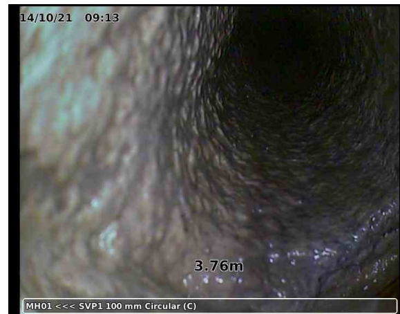
20211014-091209-snap00001.jpg, 00:01:22, 3.76 m Finish node, major connection without manhole, reference: SVP1
