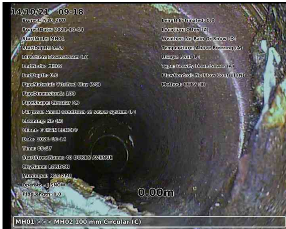
20211014-091813-snap0000.jpg, 00:00:00, 0.00 m Start node, manhole, reference: MH01
