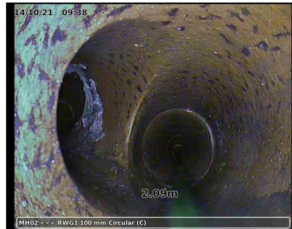
20211014-093650-snap0001.jpg, 00:00:41, 2.09 m Junction at 9 o'clock, diameter: 100mm, RWG2 - FRONT RWDP
