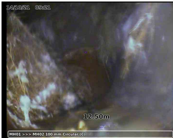
20211014-091813-snap0001.jpg, 00:02:59, 12.50 m Finish node, manhole, reference: MH02, INTERCEPTOR MH FRONT
