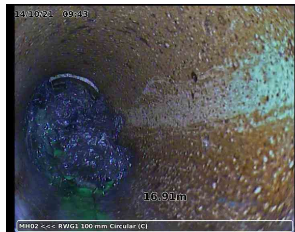
20211014-093650-snap0004.jpg, 00:04:56, 16.91 m Survey abandoned, MASS OBSTRUCTION
