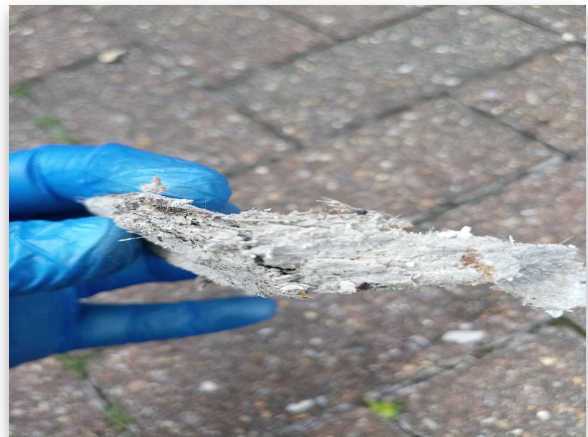
Fig 4.4: Potential asbestos containing material
