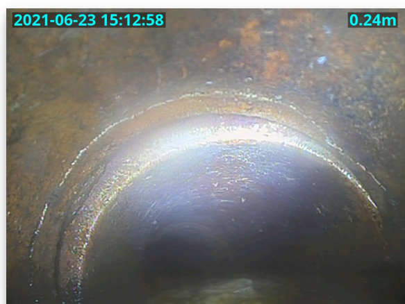
Fig 3.3: Line 3, joint displacement
