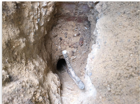
Fig 2.2: Trial Hole 3 Footing
