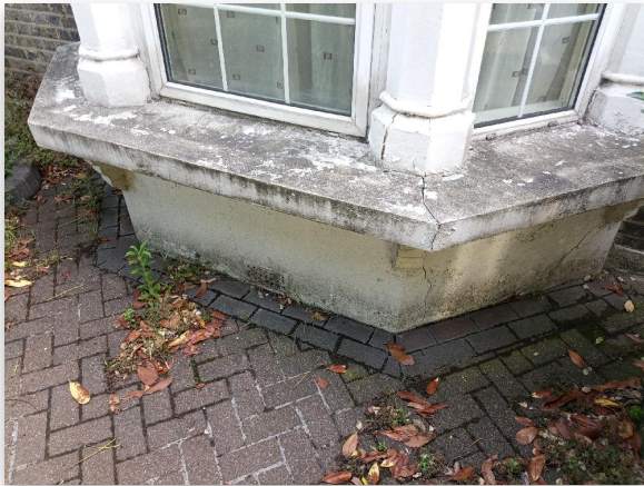
Fig 1.1: Trial Hole 1 Location
