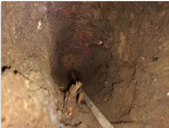
Fig 1.3: Trial Hole 1 Footing
