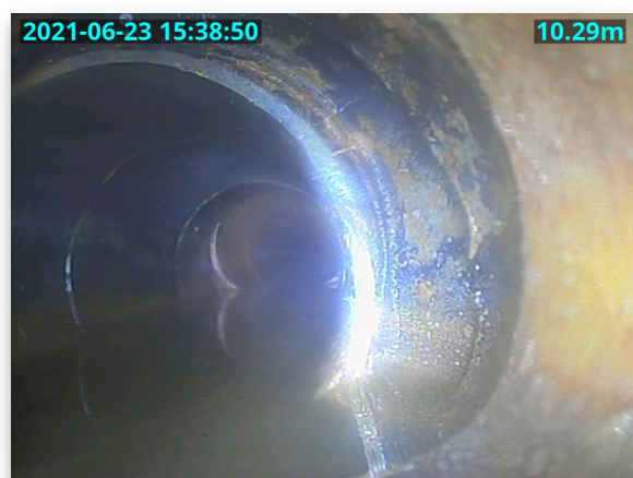
Fig 3.4: Line 4, joint displacement
