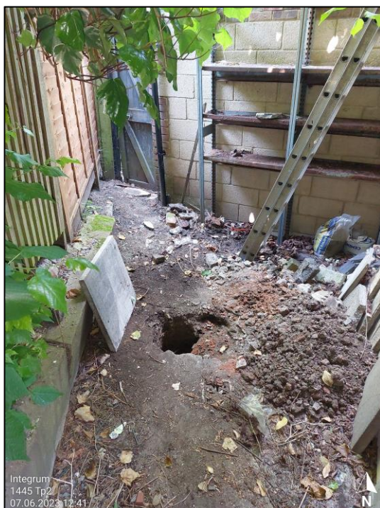
Figure 7 & 8 (below): TP2 with sparse multiple small roots <10mm \varnothing
