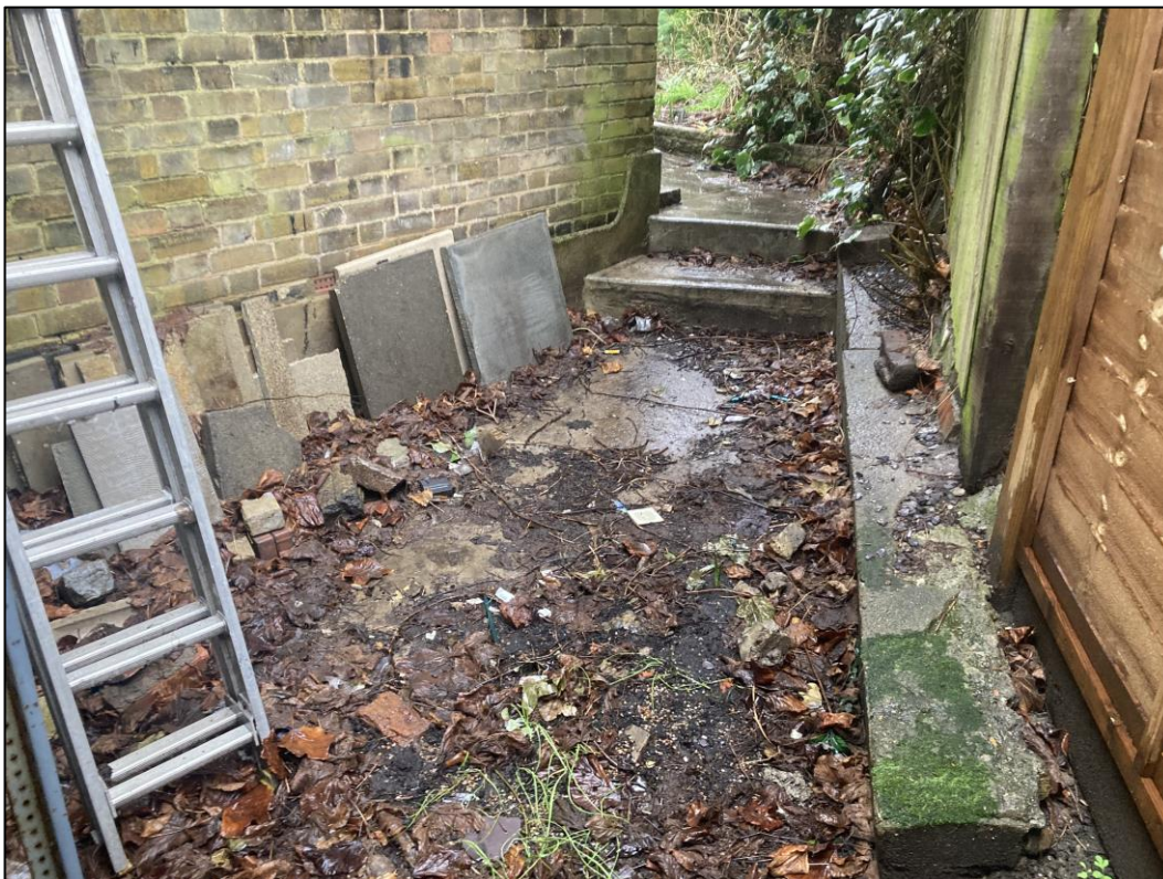
Figure 2 (left): photo showing existing hardstanding, building and level changes between the offsite tree stems and the proposed area of development which gives rise to unfavourable rooting conditions which will have likely suppressed the development of substantial rooting systems but creates difficulty in amending standard RPAs.
