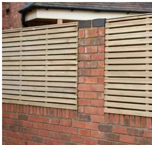
SLATTED TIMBER FENCE EXAMPLE
