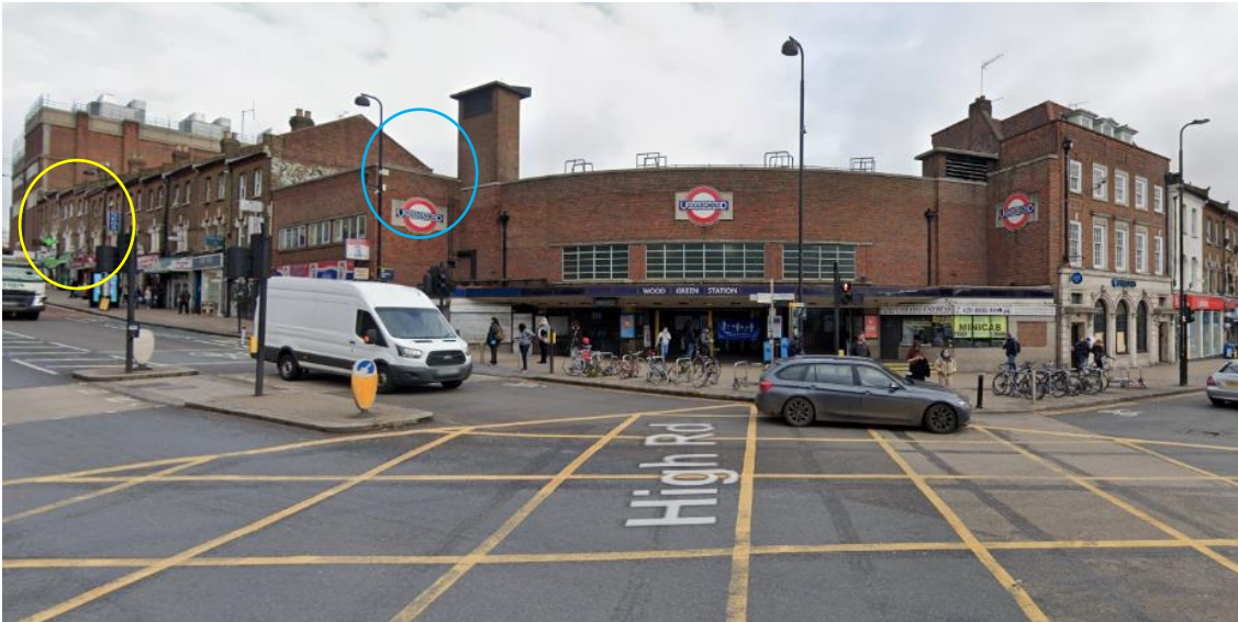
Figure 3: Front view of Wood Green Underground Station. Note that the proposed Mansard Roof Extension would not be visible from Street Level. Also note 212-214 High Street (circled in yellow) and its more prominent and elevated position on the road, with the extension being dominant on top of the hill compared to the proposal. Also note the level viewpoint of the gable end of 196 High Road and the station referenced in Paragraph 5.7 above.
