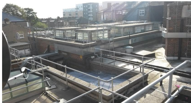
View from the rear window to roof of the underground station.
