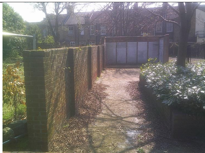
View looking south towards western part from north west corner of eastern part
