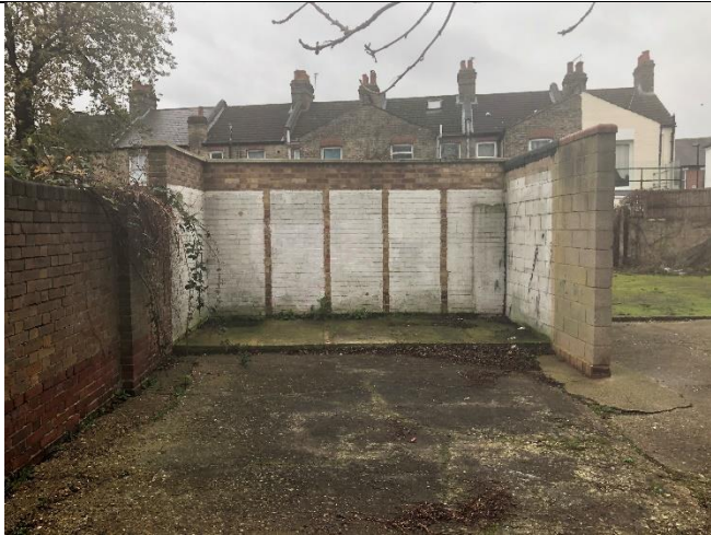
View South into brick structure in middle of Site
