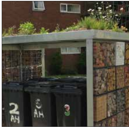
Green roof to bin store
