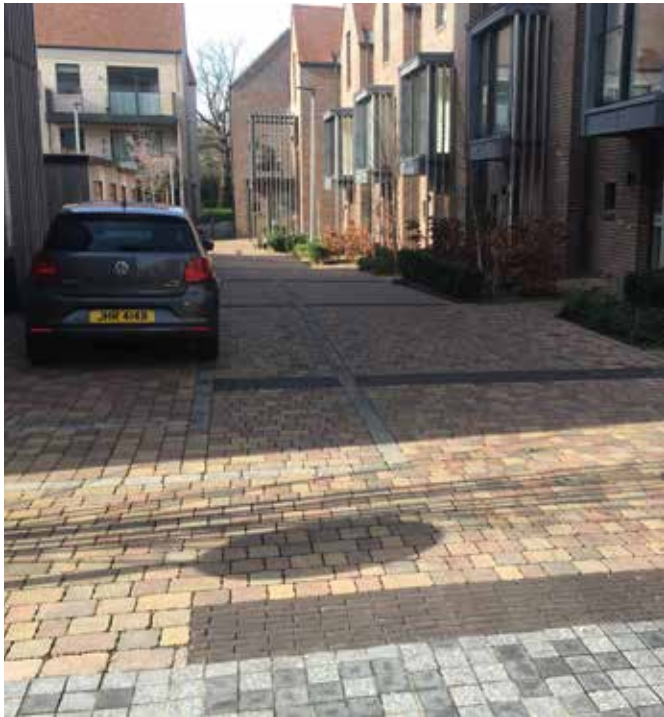
Shared surface with various colours to delineate carriageway and parking
