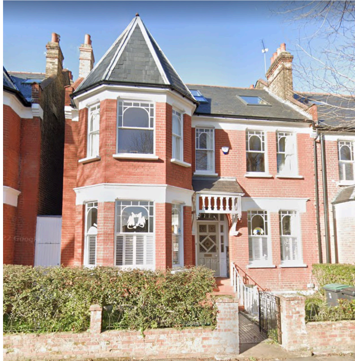
183 Mount View Road, Stroud Green, N4 4JT Front Elevation (image source: Google street view)
