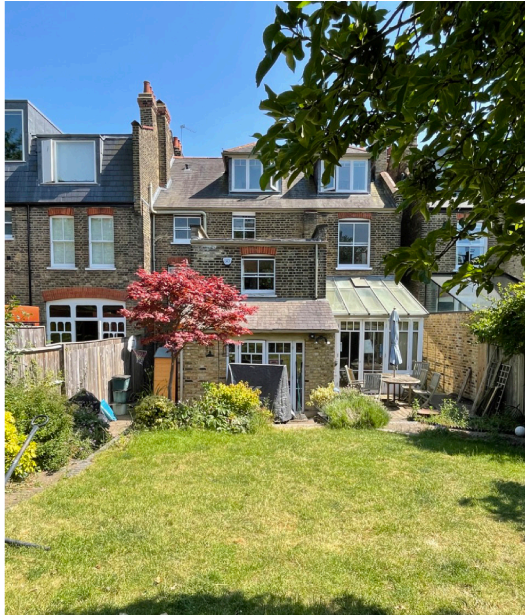
183 Mount View Road, Stroud Green, N4 4JT Rear Elevation
