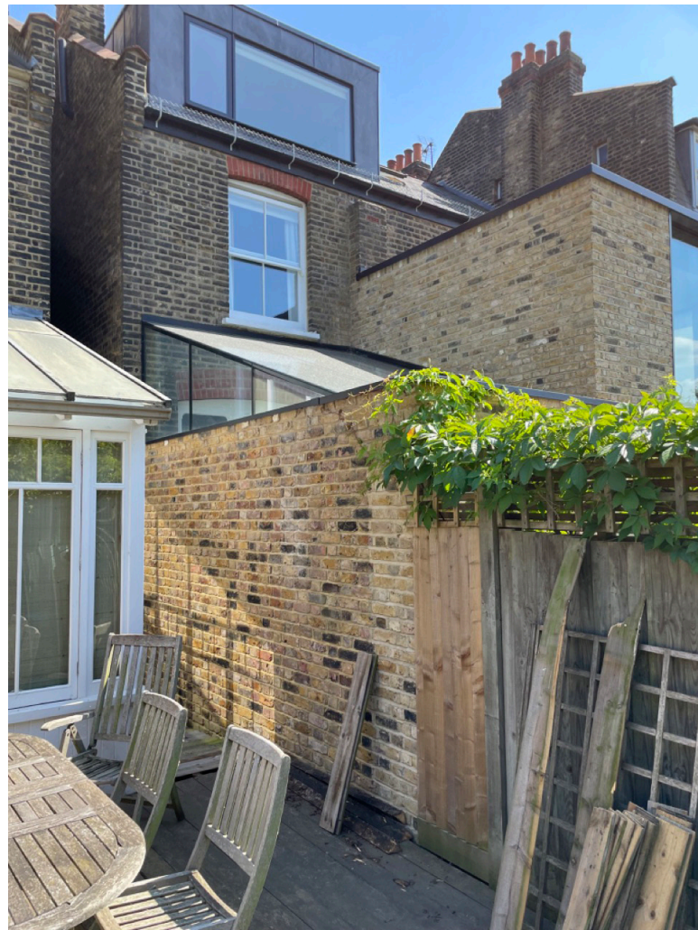
Rear elevation detail Adjoining wall and brickwork New extension sitting just under 1st floor
