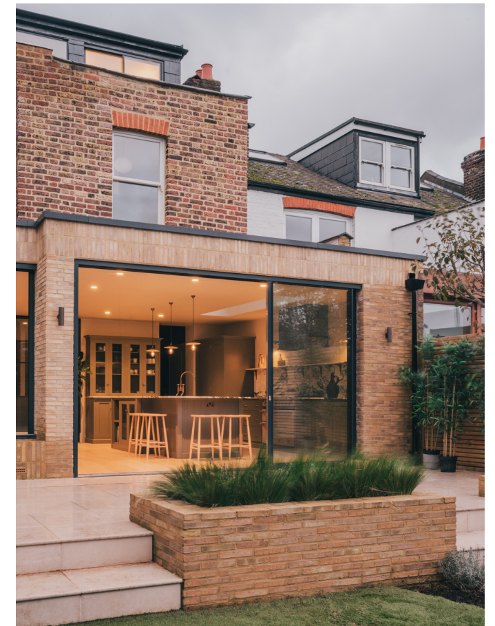
Pale brickwork to compliment existing brick facade
