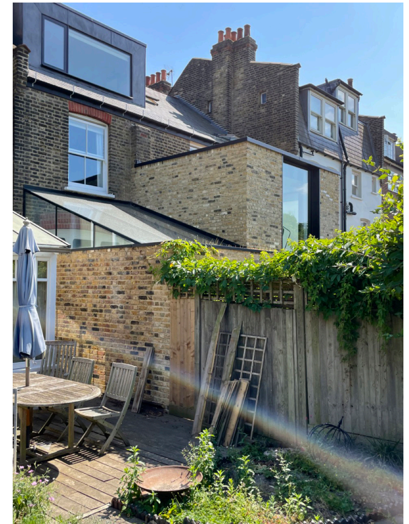
Rear elevation detail Two-storey extension New extension sitting just under 1st floor window
