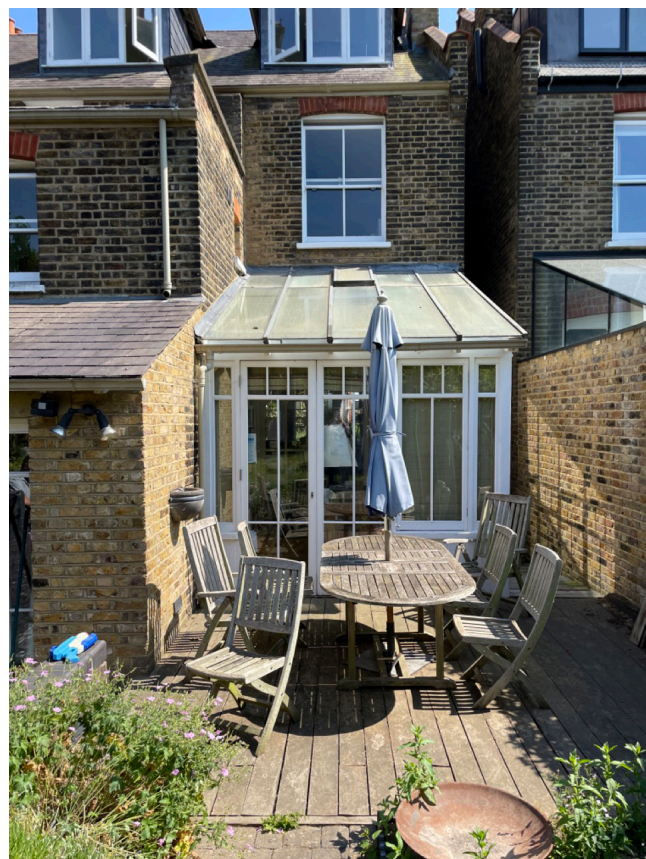
Rear elevation detail Existing Conservatory
