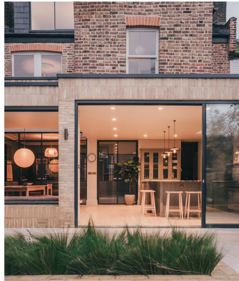
Pale brickwork to compliment existing brick facade
