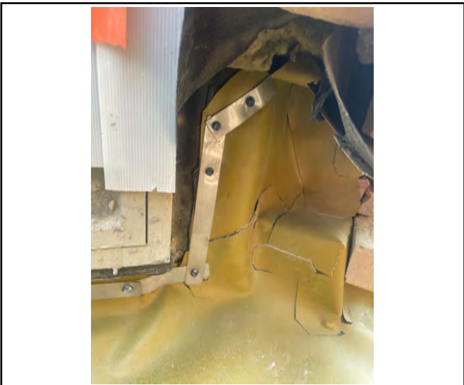
The sealed membrane into the
