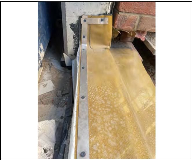
The sealed membrane into the
