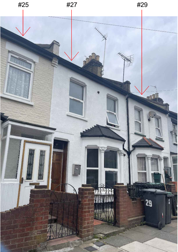
BOUNDARY CONDITIONS BETWEEN NUMBERS 27 AND 29 AT REAR
