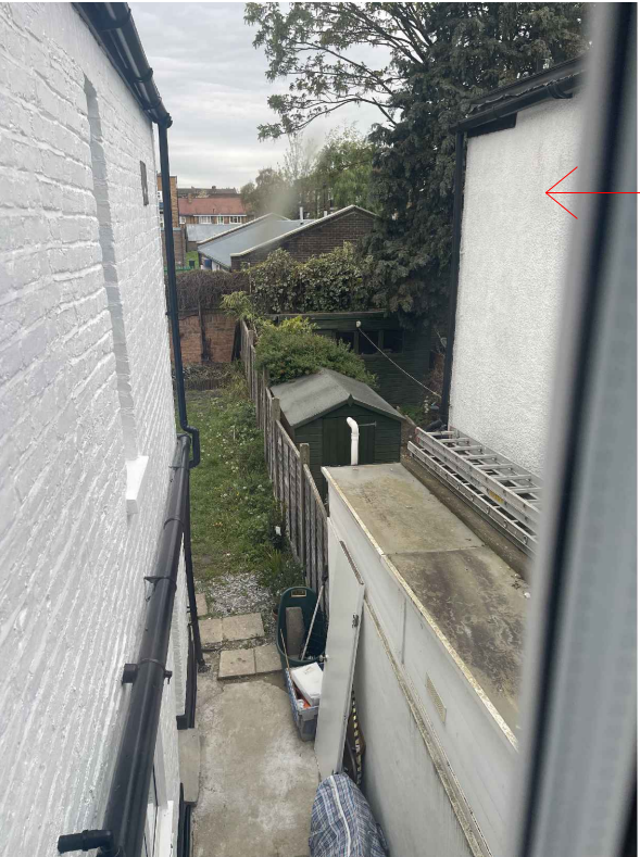
BOUNDARY CONDITIONS BETWEEN NUMBERS 27 AND 29 AT REAR
