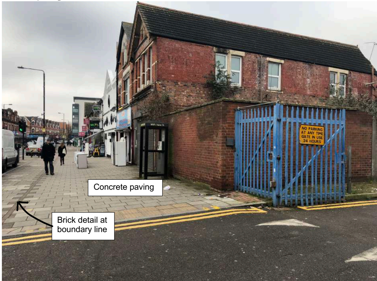
Photograph outside 306 West Green Road prior to demolition
