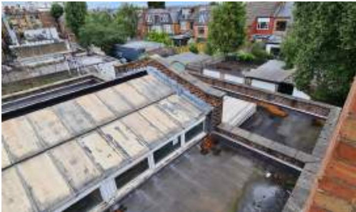
3. Rooftop View to North
