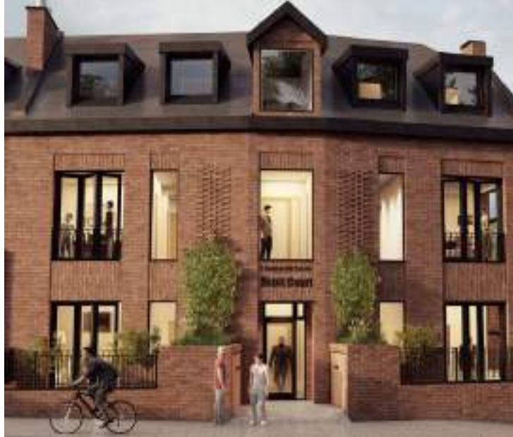
Soldier Course Brickwork Dudden Hill Project
