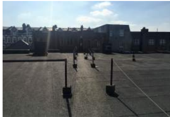
Rear Roof Level Looking North
