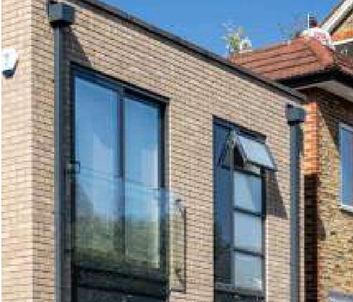
Aluminium Windows and Concrete Copping Kenilworth Road Project
