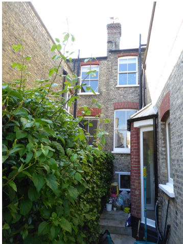
View from the rear (North)
